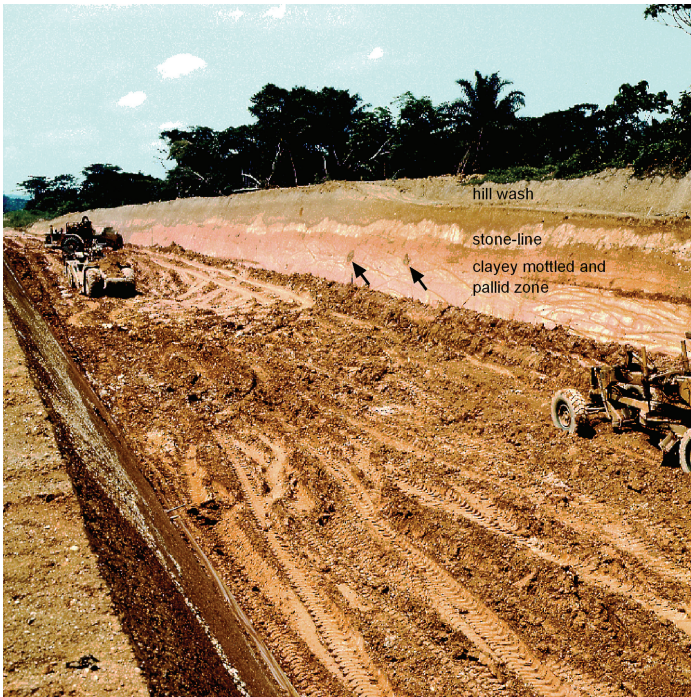
Figure 7. Road construction works under recent rain forest cover at the Osokari field site in the eastern Congo basin with fossil tree trunks (arrows) within the mottled- and pallid zone below a thick undulating stone-line that possibly marks the Pleistocene–Holocene transition (Photo: J. Runge, 1992).
