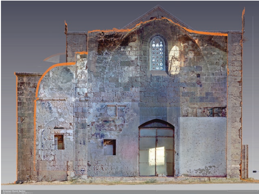
Fig. 1.6 Laser imaging of the Armenian Church: Section. Courtesy of Solvotek
