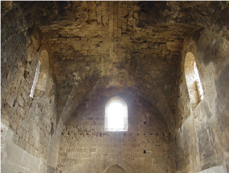
Fig. 6.7 Famagusta, Armenian Church, vault toward west
