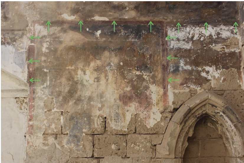
Fig. 12.2 North wall—Detail with the Baptism and the Imago Pietatis panels on the lower register. Arrows indicate the direction of overlap of plasters
