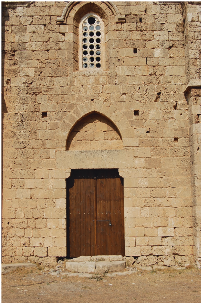
Fig. 12.3 New door, fitted in 2014
