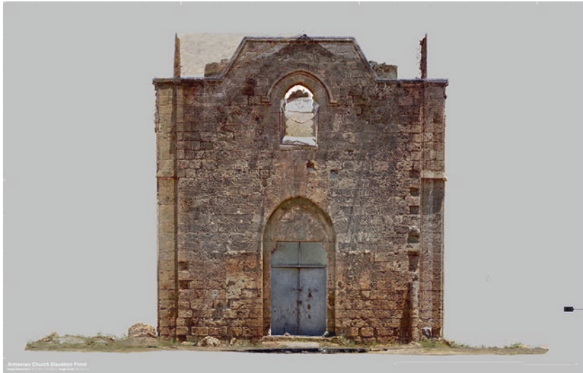
Fig. A.3 Exterior scan of western façade of the Armenian church, Famagusta
