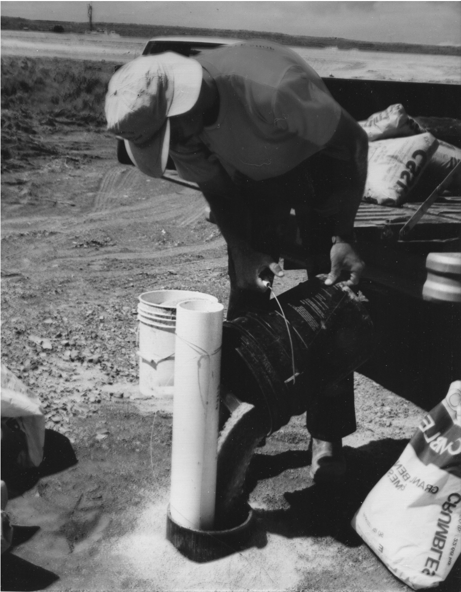
Figure 8.7. The addition of grouting materials to a borehole (U.S. DOE-INEL photograph).
