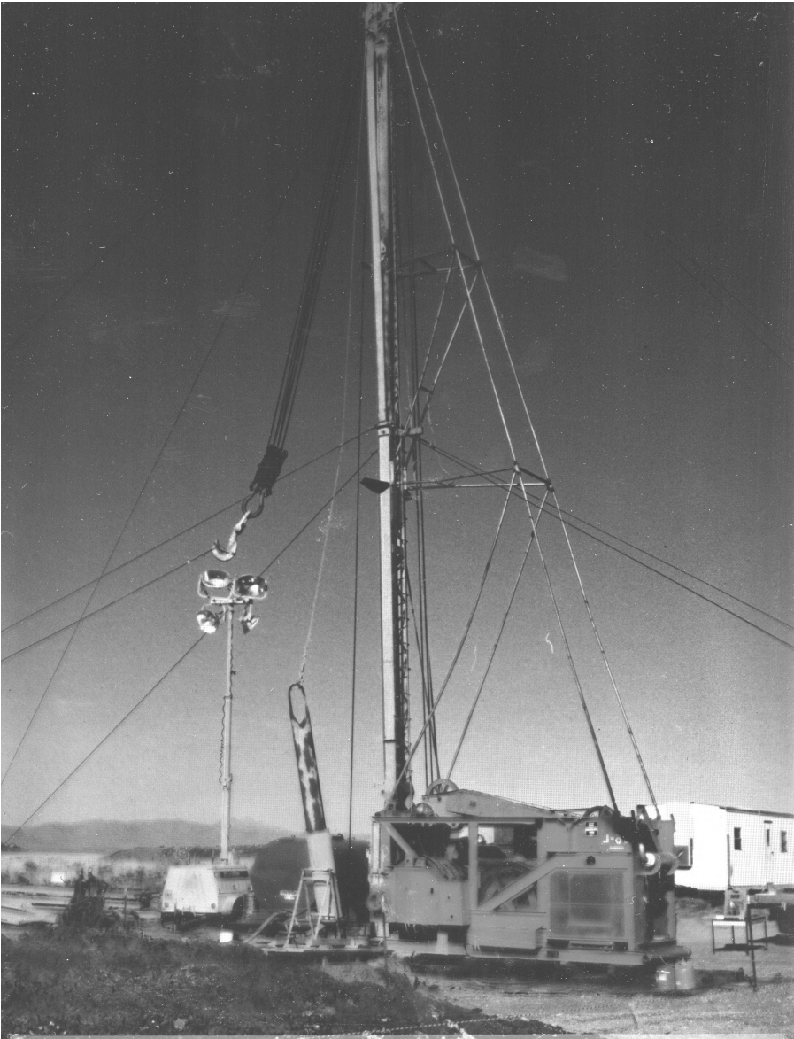
Figure 8.2. A cable tool drill rig (U.S. DOE-INEL photograph).
