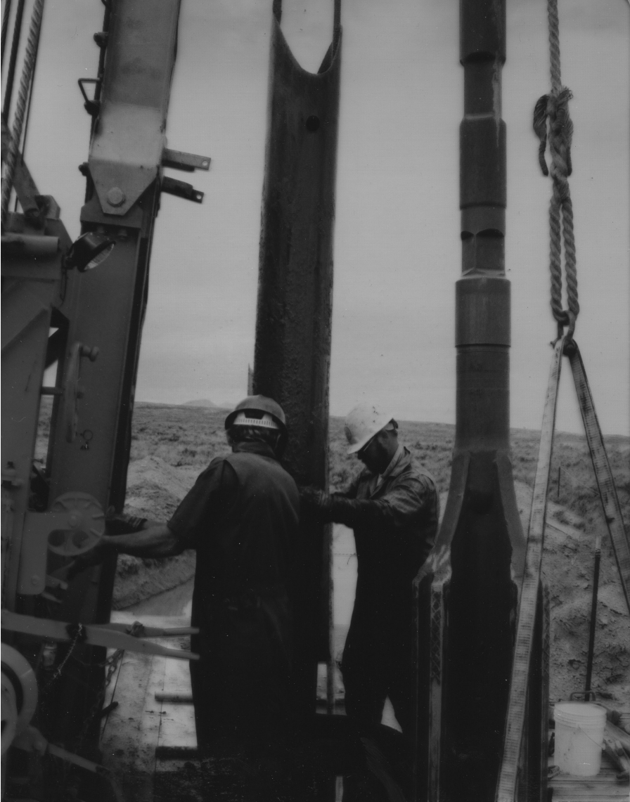
Figure 8.3. A cable tool drill bit and bailer (U.S. DOE-INEL photograph).
