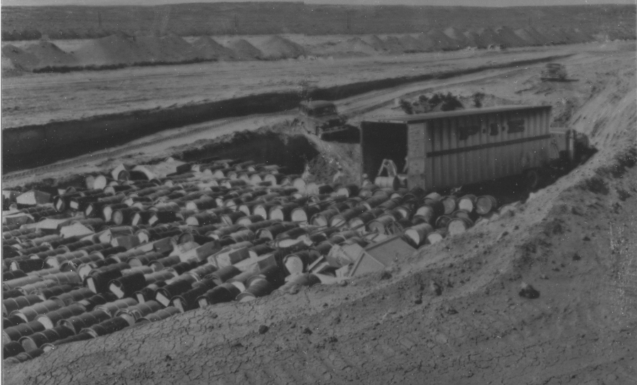
Figure 8.14. Disposal of radioactive waste at the INEEL (U.S. DOE-INEL photograph).
