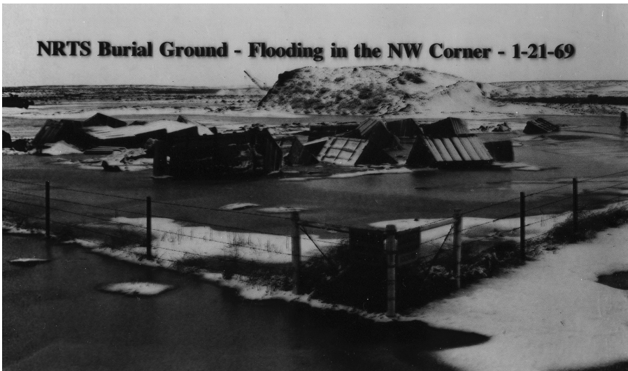
Figure 8.15. Flooding of the waste site in 1969 (U.S. DOE-INEL photograph).
