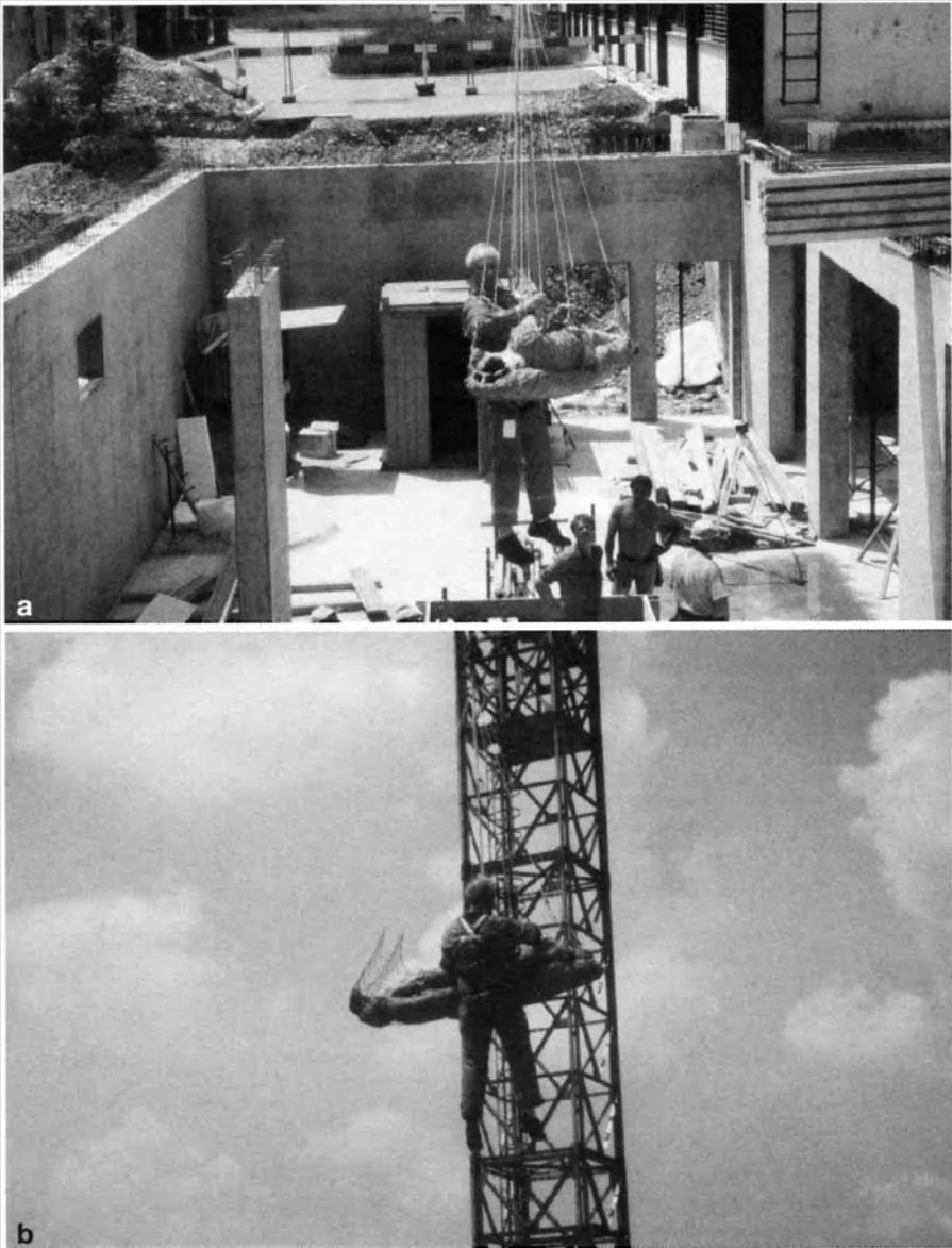
Fig. 5a, b. Use of a crane to remove a building worker
