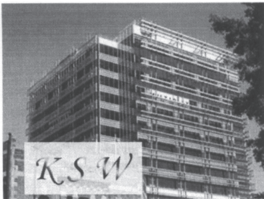
Figure 29-1. King Street Wharf in Sydney, Australia, uses Web services to analyze and manage multiple utility systems.
