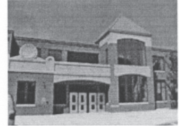
Built in 2001, this 190,000 sq.ft. middle school has an Energy Star rating of 32.
