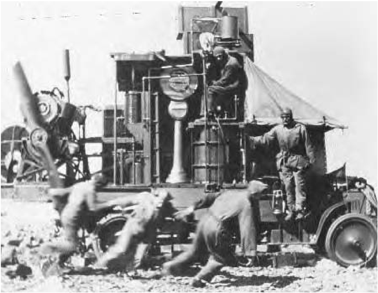
Aircraft engine developments took a great deal of time, and the superchargers that enabled the B-17s and B-24s to live over Germany derived from these early experiments with Sanford Moss's supercharger on a Liberty engine. (Walter J. Boyne)
