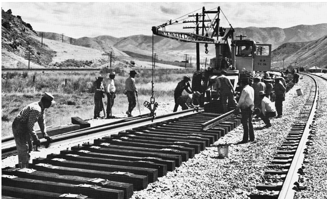
Men and machine lay railroad tracks. A common alloy of manganese, ferromanganese, is contained in the steel used to produce railroad tracks. GALE GROUP.
