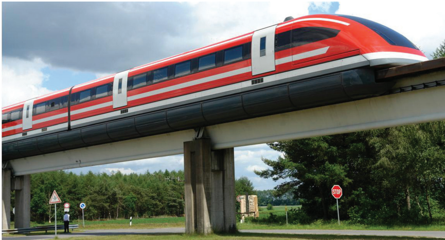
Fig. 8.9 Transrapid 08 . Photo courtesy of Thyssen Transrapid System, GmbH, München, Germany.
