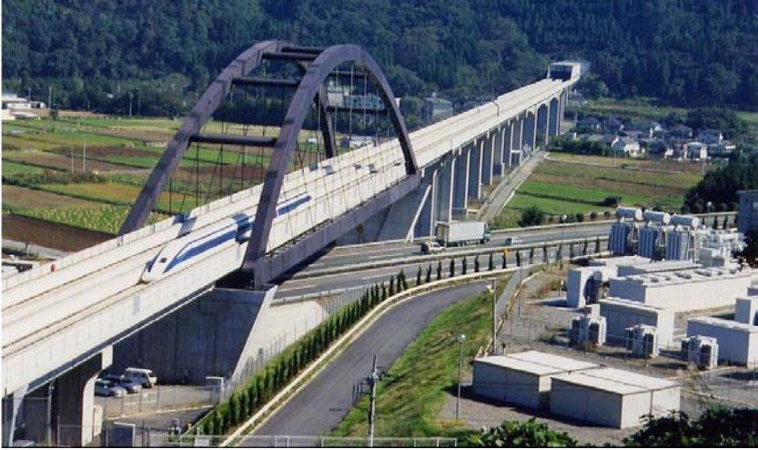
Fig. 8.13. (see color insert.) Yamanashi Maglev Test Line: Ogatayama Bridge over the Chuo Expressway. Courtesy of Central Japan Railway Company and Railway Technical Research Institute, Tokyo, Japan.
