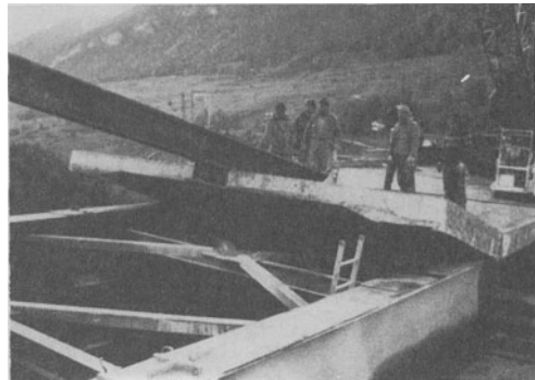
Fig. 15, Demolishment of the old deck
