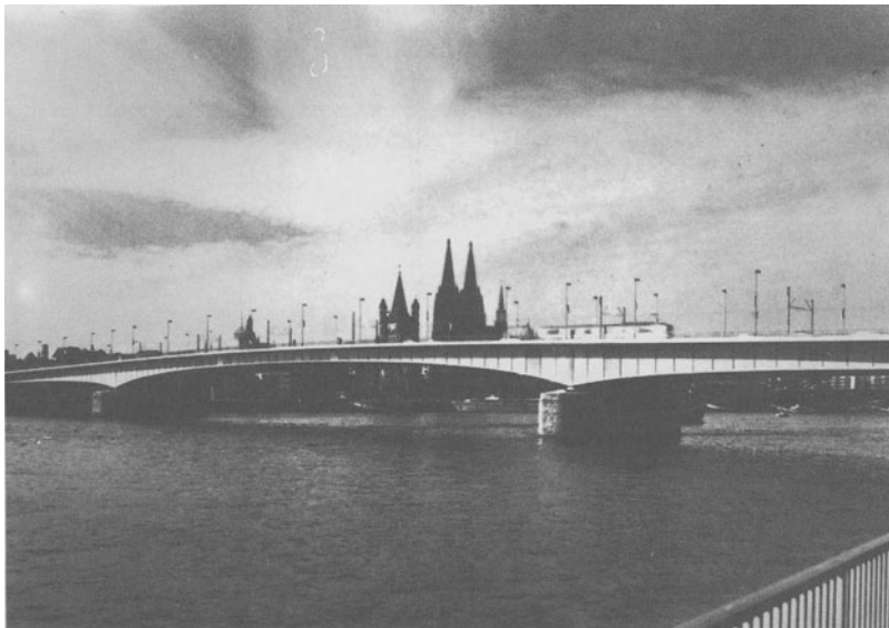
Fig. 10: View of the Rhine Bridge Cologne-Deutz
