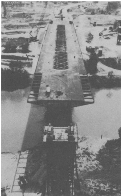
Fig.4a: Indiano Bridge (Florence) during deck erection by longitudinal launching.
