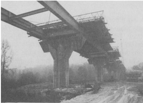
Fig. 12, Bridge over the river Oise (F) with movable scaffolding
