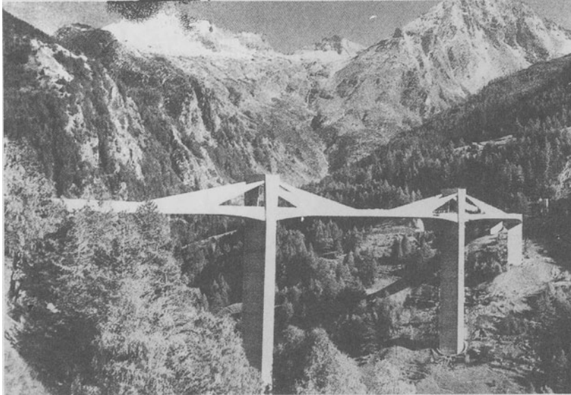
Fig. 13: The Ganter Bridge on the Simplon Pass road against the sunlight
