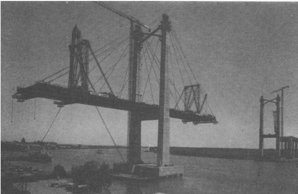
Fig.6: Zarate Brazo Largo Bridges during erection.
