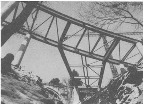
Fig. 7, Maladeire Bridge (CH)
