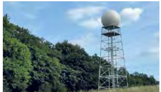
Figure 4.4 Operational radars are housed within a dome. This radar is at Dean Hill, and is part of the UK operational radar network. (Photo: Met Office.)
