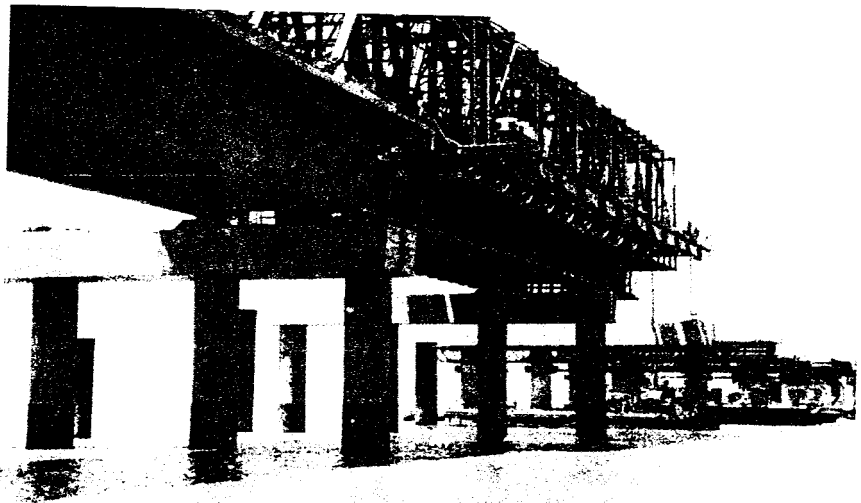
Figure 10.13. Overhead gantry for in situ beam-and-slab deck. Reproduced courtesy of Hyder Consulting Ltd. Copyright reserved.
