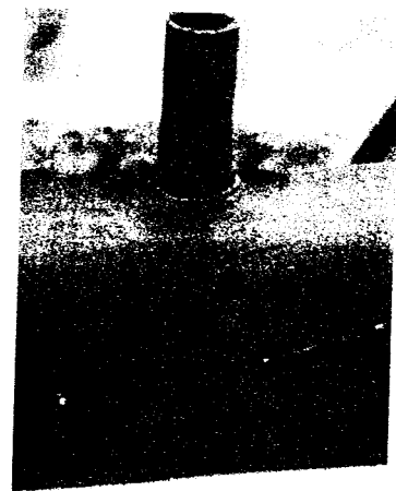
(iii) HDPE external duct
