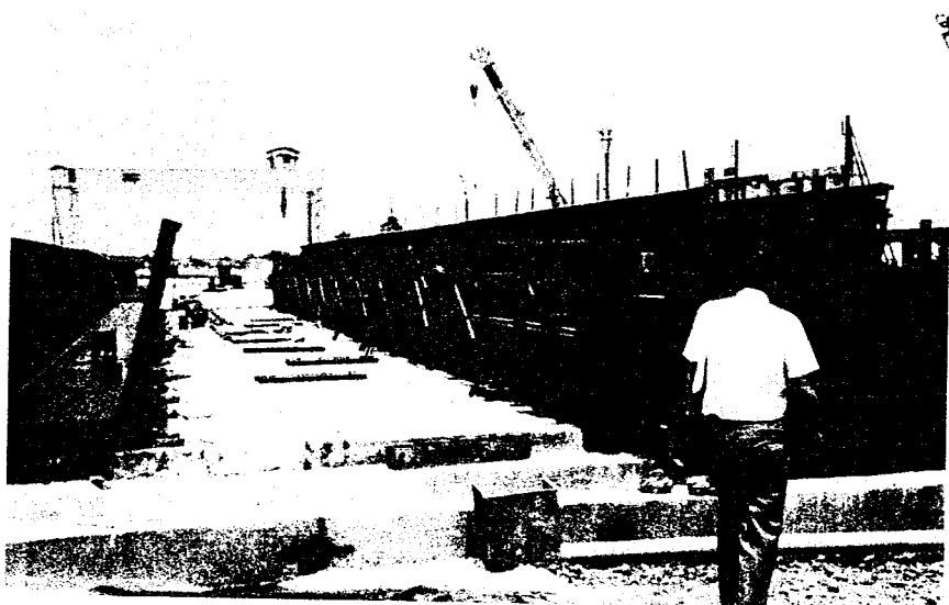
Figure 10.16. Shutter with strands anchored at ends.
