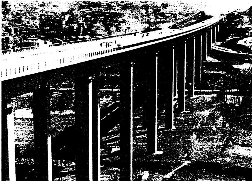
Incrementally launched box girder bridges
