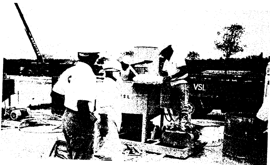
Figure 4.3. Grout mixing equipment. Reproduced courtesy of Louise Smith. Copyright reserved.
