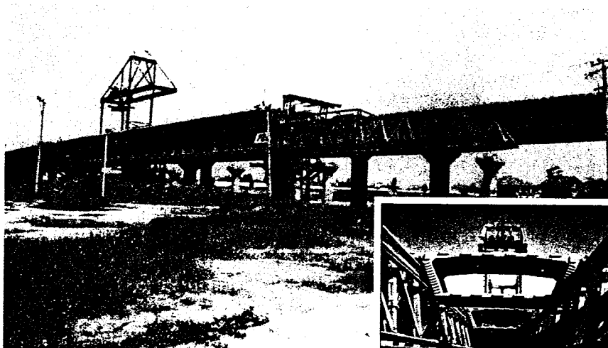
Figure 13.44. Underlung truss for span-by-span erection.
