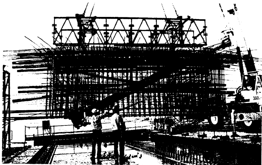
Figure 16.14. Prefabricated reinforcement cage. Reproduced courtesy of VINCI Construction Grands Projets. Copyright reserved.
