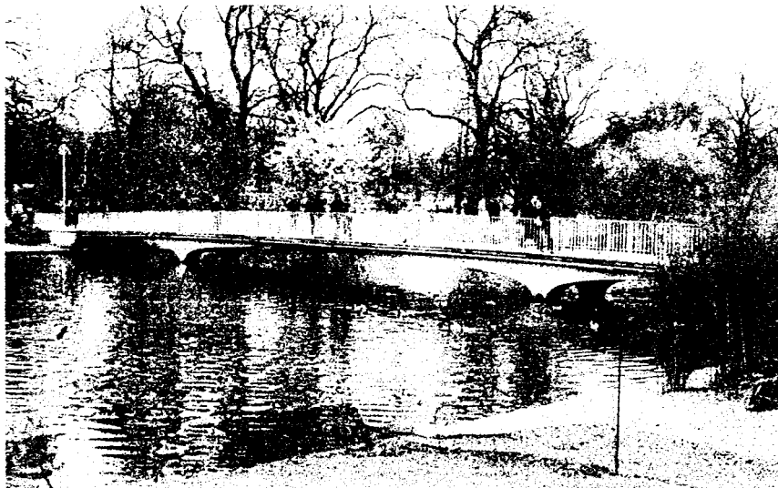
Figure 1.14. St James's Park Footbridge, England.
