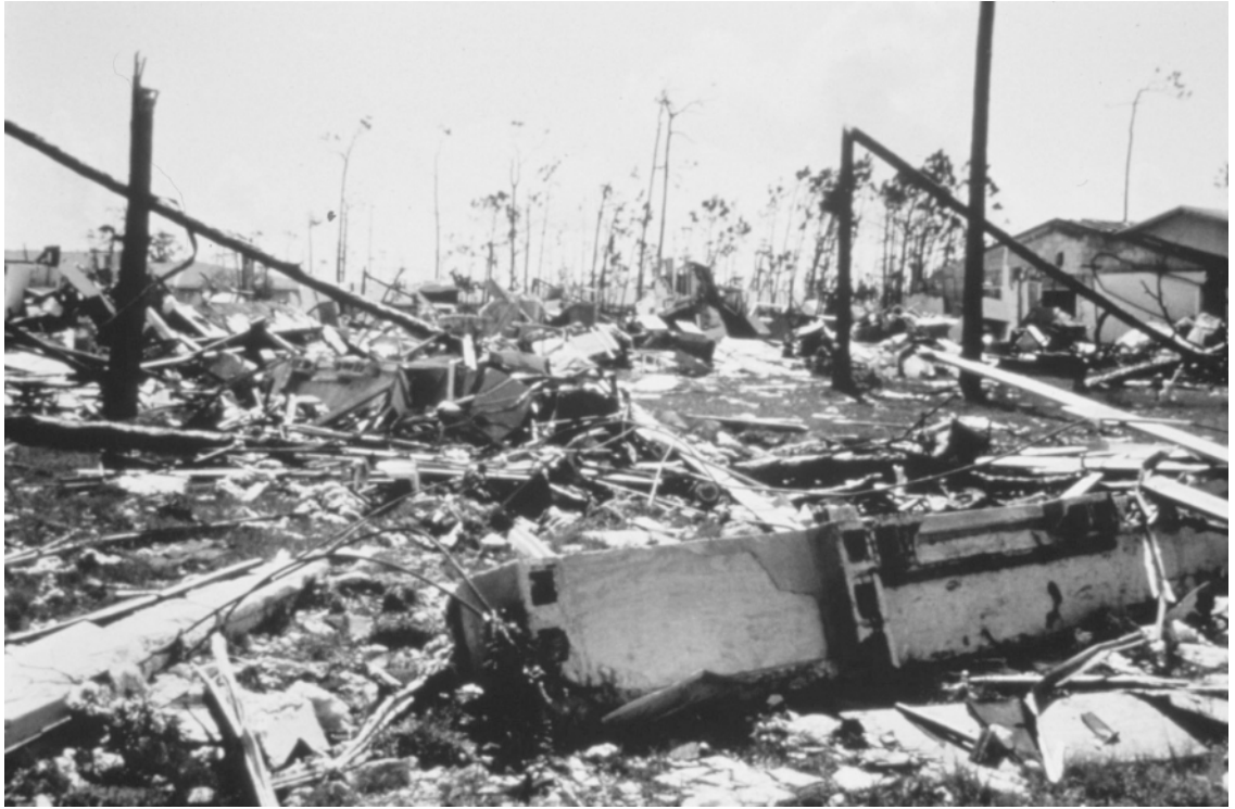
Plate 22 Ground view of the devastation caused by Hurricane Andrew in Pinewoods Villa, southern Florida, 23–24 August 1992 (courtesy of NOAA, NOAA Photo Library Historic NWS Collection wea 00534).
