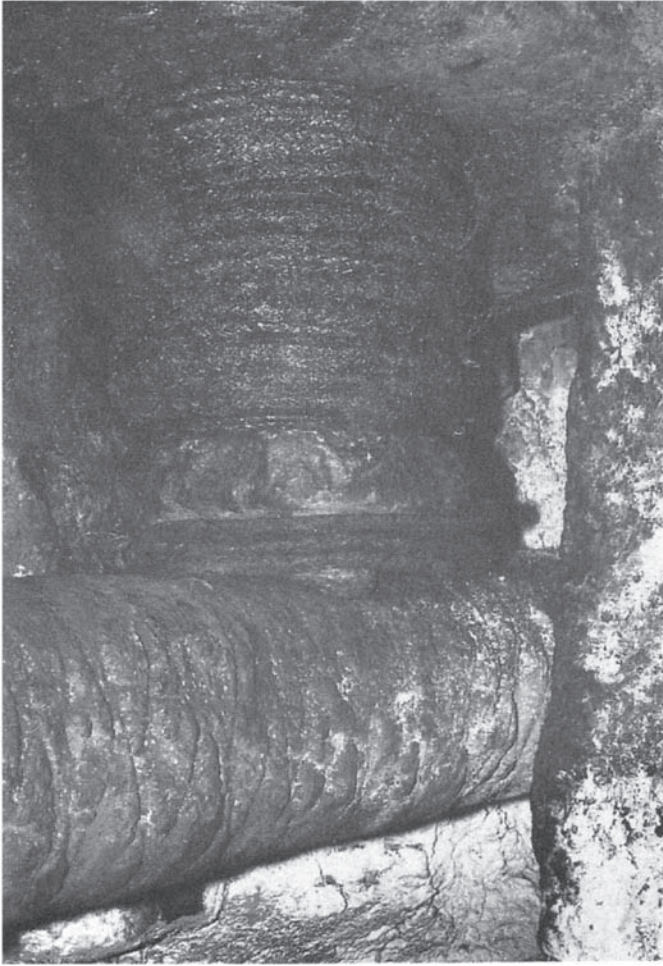
Figure 9.8 Baskets of pulped olives under pressure below the beam of a lever press still in use in 1987. (Douiret, S. Tunisia.)
