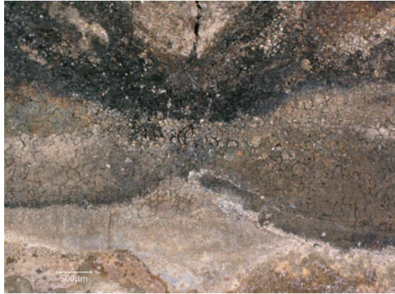
Fig. 11 IGA-like features were observed at one of the crack tips
