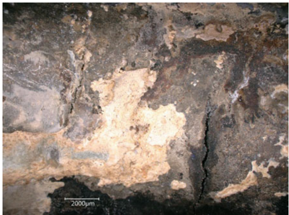
Fig. 10 Higher magnification view of the tube #17 cracks
