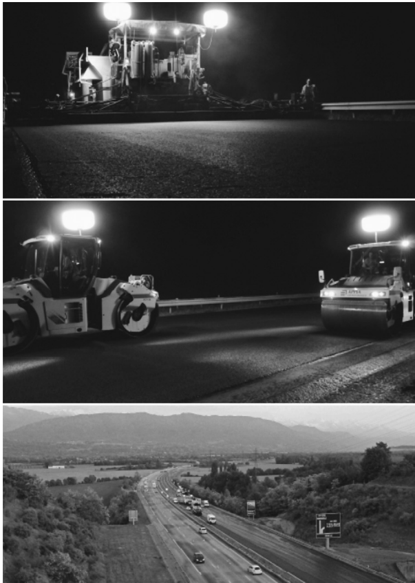
Figure 14.18 12,000-t GB5 ® 0/14 roadwork on the French A43 toll highway (AREA network, Chignin-Francin section) in the alpine area. Budillon aggregate, 15% RAP, and PMBs Biprène ® 41 and Orthoprène ® were used.
