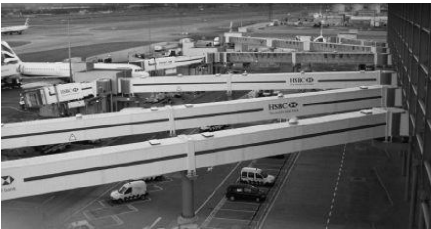
FIGURE 3.4 Typical European contact position: long distance between building and aircraft featuring a long bridge over road and parking spaces. ( Source: London/Heathrow terminal 5.)
