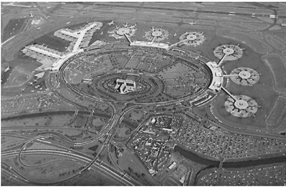
FIGURE 14.7 Decentralized passenger buildings at New York/Newark Liberty. ( Source: Port Authority of New York and New Jersey.)
