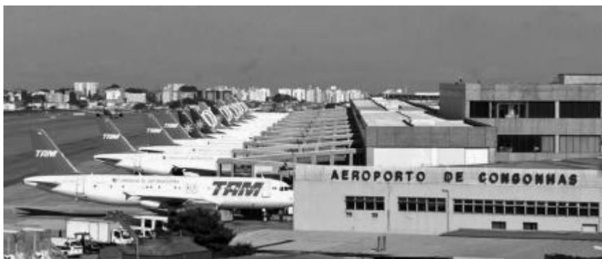
FIGURE 3.3 Aircraft connecting directly to passenger building. ( Source: Aeroporto de Congonhas.)
