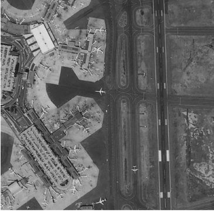
FIGURE 9.22 The “horseshoe” apron between passenger buildings B and C at Boston/Logan and the entrance to that area. ( Source: Massport.)
