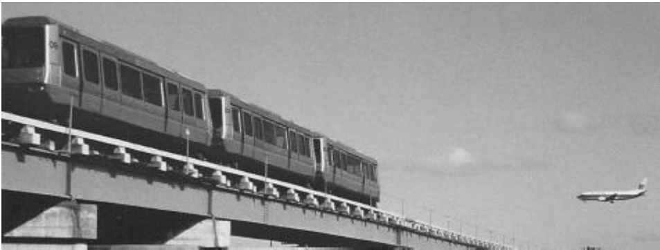
FIGURE 17.7 Siemens VAL at Chicago/O’Hare. ( Source: Harley Moore, Lea+Elliott, Inc.)
