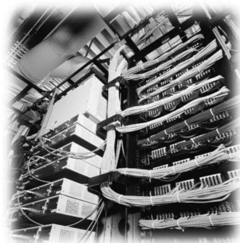
FIGURE 18.4 Lucent SYSTIMAX GigaSPEED Installation, rear angle view of patch-panel rack. (Copyright © 1999, Lucent Technologies, used by permission.)
