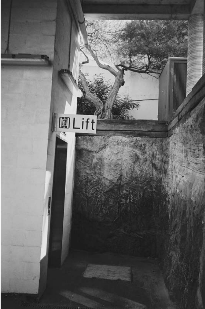
Figure 6.1 An access elevator at Waverton Station, northern Sydney. Local residents agitated for elevators when the commuter train system proposed renovations to the station along historic lines. This represents both a good technical solution to access problems and an unwelcoming signifier, in that the layout and the rock-cut walls combine to create a dungeon-like feeling. Photo by Rebecca Dobbs.
