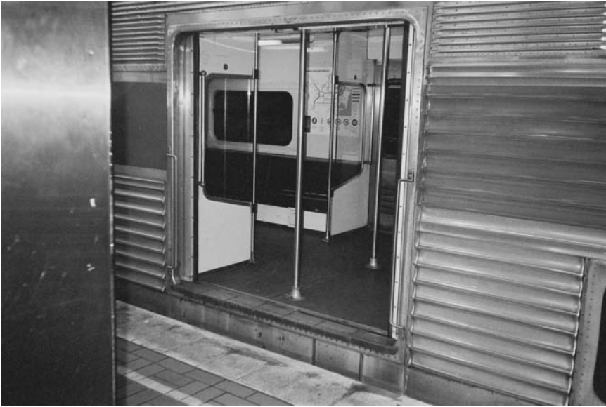
Figure 6.2 Step up from platform to train in Sydney CityRail station. This step is obviously a problem for many disabled people. Only a few (generally newer) stations in Sydney are without this height differential, even though there is no obvious reason for reproducing this disabling design. Photo by Rebecca Dobbs.
