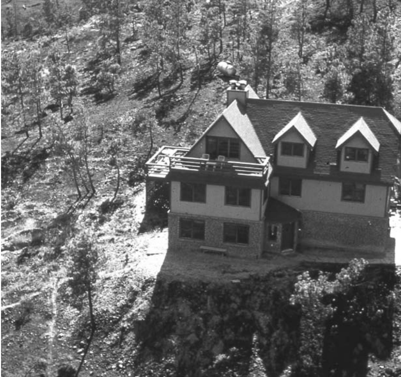
Figure 5.4 An exurban home saved by firefighters, Black Tiger Fire, Boulder County, Colorado, 1986. Development in the “wildland-urban interface” means that firefighters must not only suppress natural fires that might eventually move into the exurban zone, but also expend greater efforts to protect isolated structures. ( William Travis photograph. )
