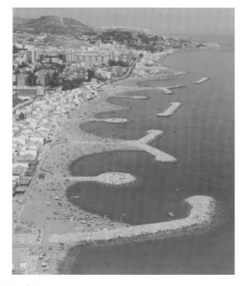
Fig. 8.3. A general view of Malaga beach regeneration scheme showing rock groynes and offshore rubble mound breakwaters (courtesy Director General Ports and Coasts, Spain).
