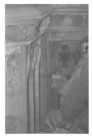
Fig. 10.10. Air abrasive cleaning in progress.
