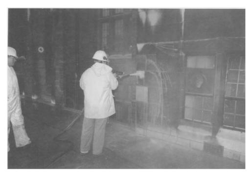
Fig. 10.7. Cleaning trials in progress on a Portland stone building.
