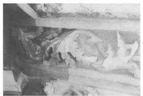
Fig. 10.13. Two views of masonry comparing cleaned and uncleaned areas.
