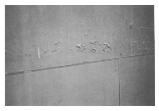
Fig. 10.6. Blistering on a limestone (Bathstone) façade in north London.
