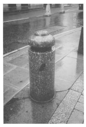
Fig. 9.28. Bollard of porphyritic Shap granite, St. Pauls, London.
