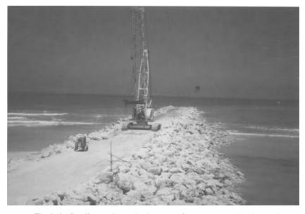
Fig. 8.19. Crestline roadway allowing access for transport and equipment.
