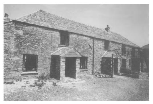
Fig. 9.21. Example of a building with a traditional metamorphic slate roof.
