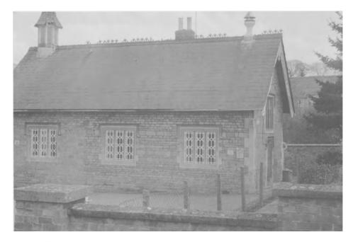
Fig. 3.3. A building of coursed iron-rich Marlstone Rock Bed from Jurassic Middle Lias near Grantham. The thickness of the stone courses is dictated by the thickness of the beds from which the stone was obtained. Since the local stone from which the building was built is not particularly durable, the dressings are of Lower Lincolnshire Limestone which outcrops about 1.5 kilometres to the south.
