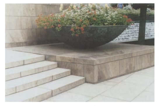
Fig. 9.29. Contrasting appearance of the same stone finished by flame texturing (steps) and polished (walls), Cabot Square, Canary Warf.
