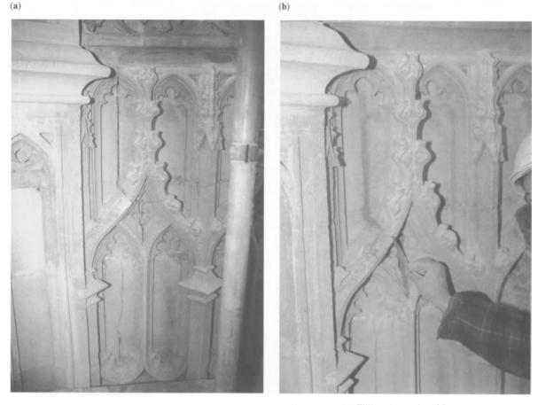
Fig. 10.23. Mortar (plastic) repairs to stone. (a) Cracks in masonry. (b) Filling the cracks with mortar.
