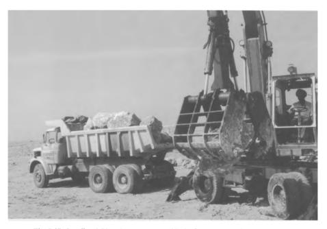
Fig. 8.17. Loading 0.75 to 3 tonne armour blocks for transportation overland.
