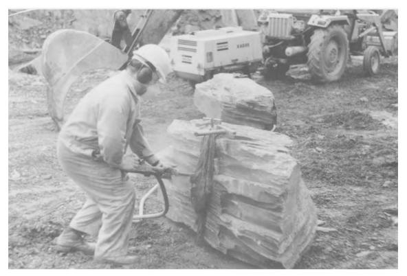
Fig. 5.26. Pneumatic top hammer drill being used to drill a hole for plug and feathers (Courtesy of Ffestiniog Slate Quarry Co. Ltd).
