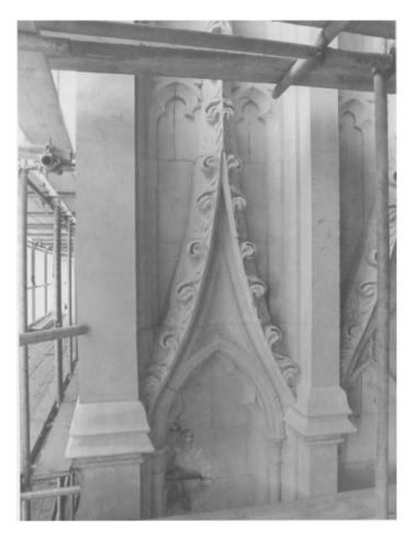
Fig. 10.3. Rusting iron cramps causing damage to stone.
