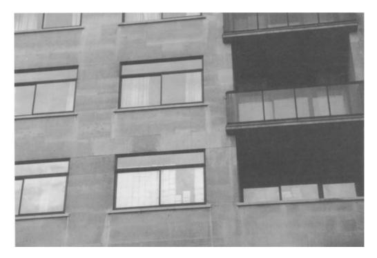
**Fig. 10.22.** The façade of this building in Knightsbridge is clad in Portland stone which has been repaired by replacement of some panels. However, they have not weathered to match the original.
