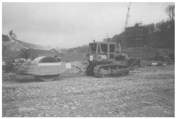
Fig. 7.15. Rock fill placement at Queen's Valley dam; compacted surface of fill.
