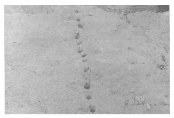
Fig. 5.38. Fracture connecting drill holes produced by hydraulic splitters (Courtesy of ARC Ltd).
