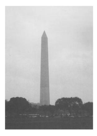
Fig. C11. The Washington Monument, 169 m high, is the tallest self-supporting masonry structure in the world (see text). It was designed by the architect Robert Mills and largely constructed by the US Army Engineers. Construction commenced in 1848 and was completed in 1885, but there was a hiatus in construction from 1854 to 1879. (*Photo: D. Newill.*)
