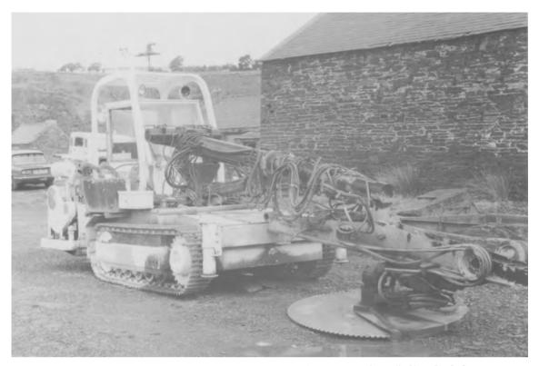
Fig. 5.32. Circular diamond saw mounted upon crawler tracks (Courtesy of Nantlle Slate Co. Ltd).
