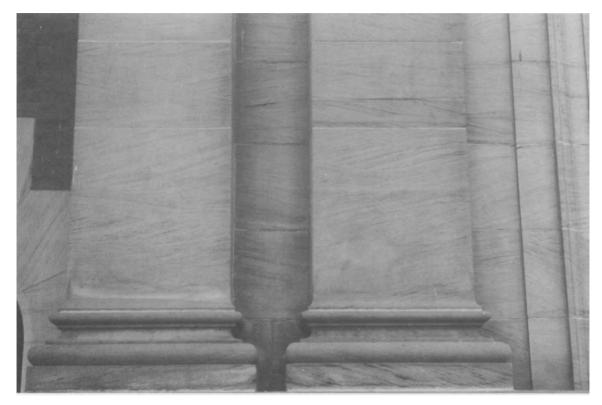
Fig. 2.47. Masonry constructed of sandstone showing evidence of current bedding (Public Library, Middlesbrough).
