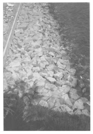
Fig. 8.7. Example of primary armour on a rubble mound coastal defence system.
