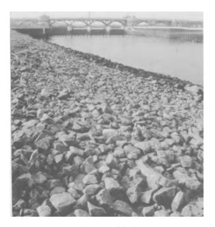
**Fig. 8.10.** Example of rip-rap used in the Tees Barrage (courtesy of Bardon (England) Ltd).
