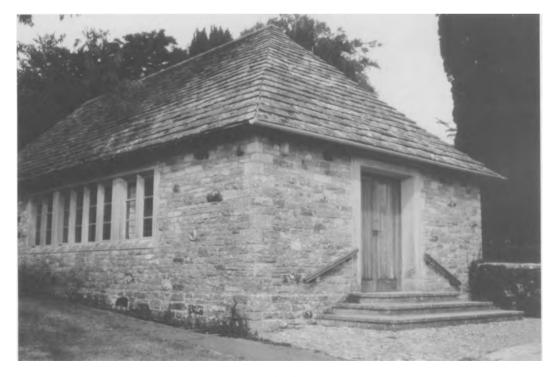
Fig. 9.20. Example of a stone tiled roof.
