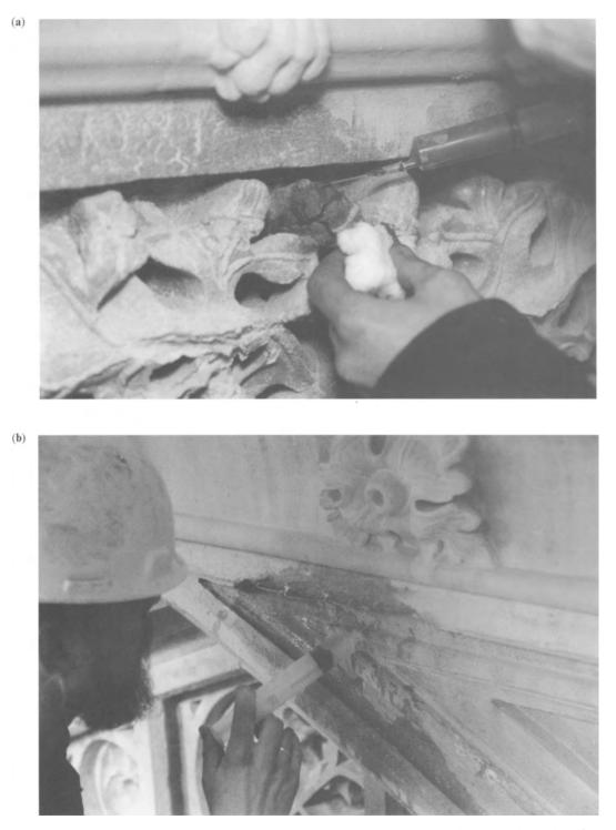
Fig. 10. 25. (a) Plastic repair using resin bound mortar. (b) Plastic repairs showing reinforcement of stone by resin injection and wire supports.
