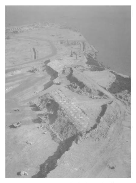
Fig. 7.20. Excavation of rock fill from blasted benches, December 1994.
