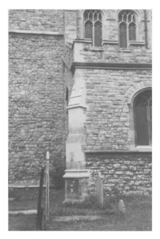
Fig. 10.19. Repairs to a buttress of All Saints Church, Fulham by replacement of stones.
