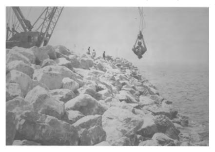
Fig. 8.20. Claw grab crane placing armourstone, Dibba Harbour.
