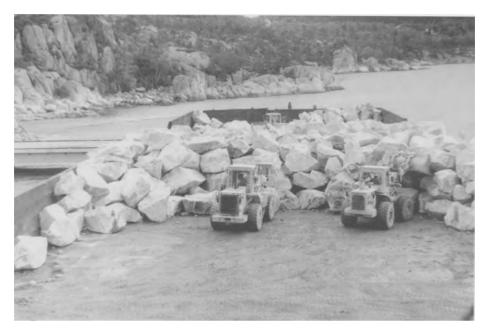
Fig. 8.16. Loading of an armourstone carrying barge, Scandinavia (photography courtesy of J.-P. Latham).
