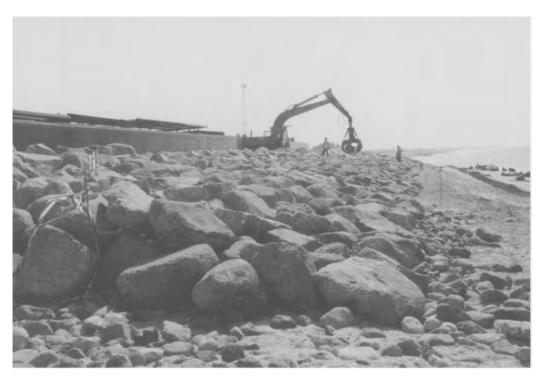
Fig. 8.21. Hydraulic claw grab placing armourstone on the Dawlish Warren coastal defence.
