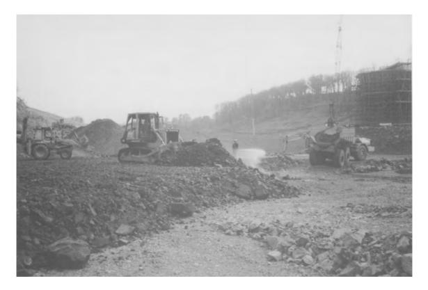
Fig. 7.14. Rock fill placement at Queen's Valley dam; pushing fill over advancing face.
