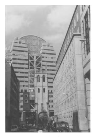
**Fig. 9.16.** Modern building with sub-frame mounted stone cladding behind an older stone masonry tower and building clad with Portland limestone.
