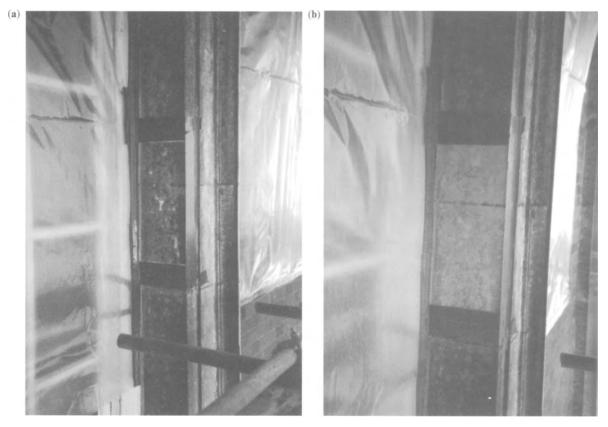
Fig. 10.8. Trial cleaning. (a) Masked cleaning trial area before cleaning using Joss system. (b) Trial area after cleaning.
