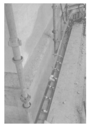
Fig. 10.9. Cleaning stone with low pressure water sprays.
