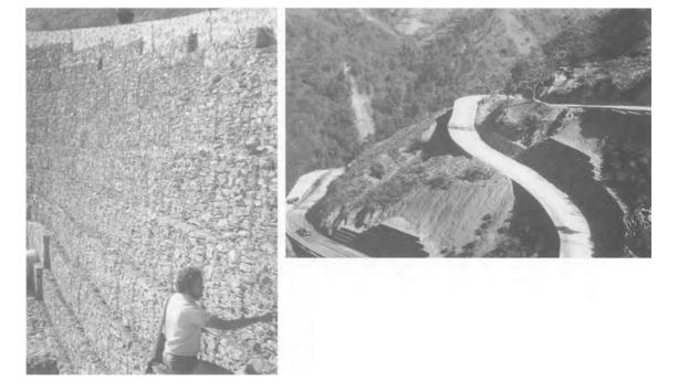
Fig. 7.5. Gabions in use for road construction (Courtesy P. G. Fookes).
