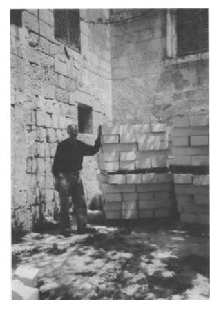
Fig. 2.18. Sawn masonry blocks of soft, cream coloured limestone, Mdina, Malta G.C.
