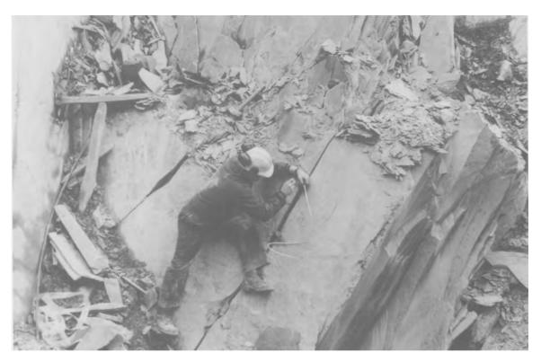
**Fig. 5.47.** Stemming being rammed into a blasthole loaded with black powder. The quarryman is lying on the cleavage plane of the slate and the hole is drilled on the pillaring plane. The safety fuse is clearly visible (Courtesy of Ffestiniog Slate Quarry Co.).
