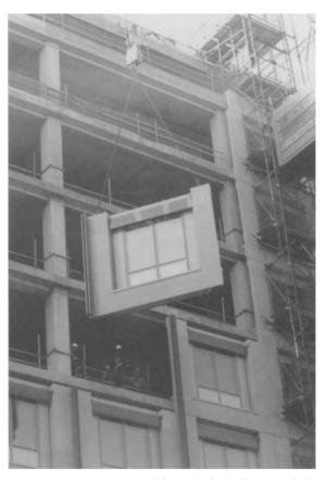
Fig. 9.17. Precast concrete sub-frame clad with limestone being lowered into position (Centre West, Hammersmith).
