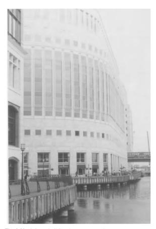
Fig. 9.30. A large building in UK unusually clad with marble (Vermont), Canary Wharf.
