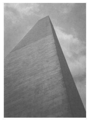
**Fig. C12.** Close-up view of the Monument. The exterior is of white marble from Maryland and Massachusetts with an interior of granite. Within the obelisk there is a shaft containing eight wrought-iron columns supporting a stairway and elevator. The slight change in colour of the marble about a quarter of the way up marks the level where construction was interrupted. (*Photo: D. Newill.*)
