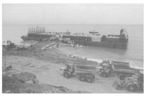
Fig. 6.7. Barge loaded with armourstone (Courtesy of Tarmac plc).
