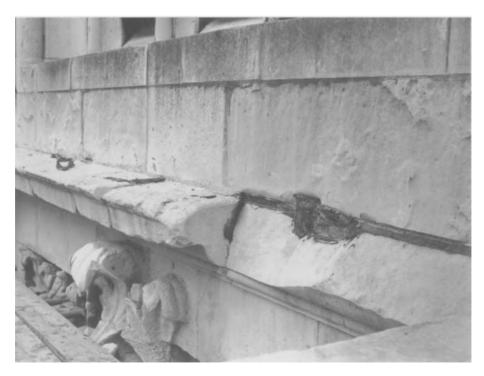
Fig. 10.2. Stone that has been broken away by the rusting and expansion of an iron cramp.
