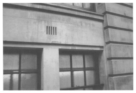
Fig. 10.21. Indentation repairs poorly carried out so that the repairs do not match the original.
