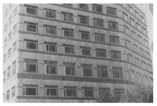
Fig. 9.31. Staining of unknown cause on one facade of a building.
