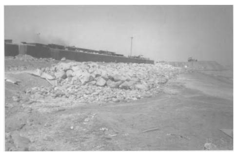
Fig. 8.9. Example of primary armouring showing the underlying secondary armour layer on a coastal defence structure.
