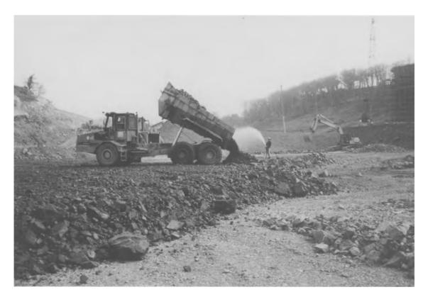
Fig. 7.13. Rock fill placement at Queen's Valley dam; dumping and watering the fill.
