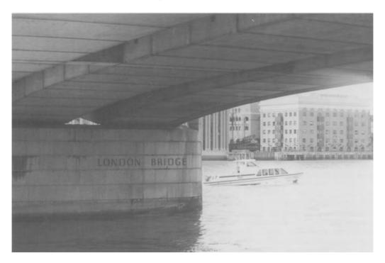
Fig. 9.26. Piers of the new London Bridge clad in Cornish granite.
