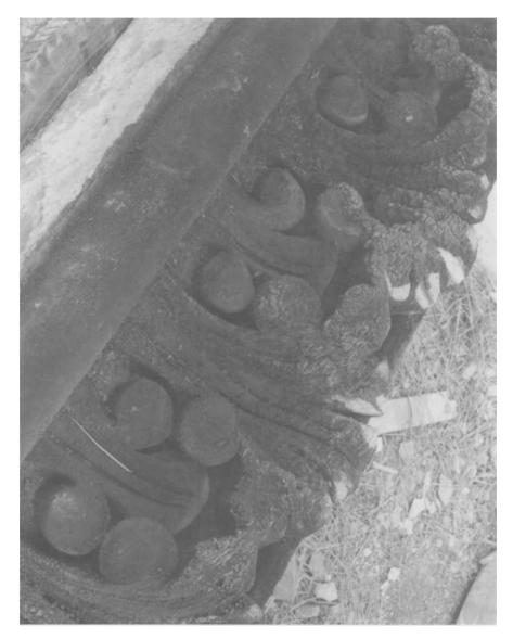
Fig. 10.4. Heavy deposits on the underside of a string course that is so badly damaged it has been cut out for replacement.
