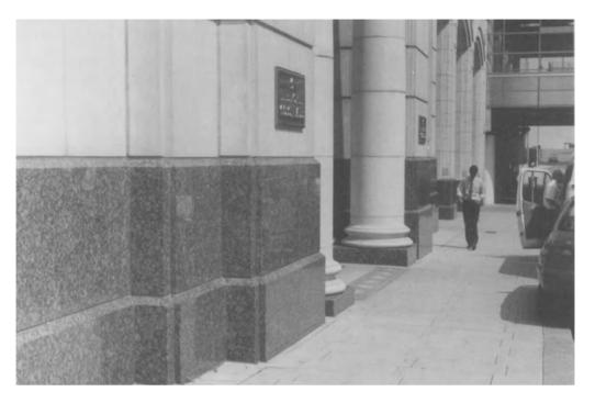
Fig. 9.22. Plinth (orbicular granite) contrasting with building facade (limestone).
