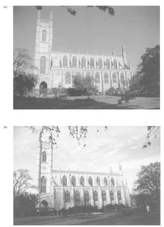
**Fig. 10.15.** (a) South elevation of St. Luke's Church, Chelsea after cleaning in 1991. (b) South elevation five years after cleaning.
