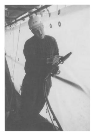
**Fig. 10.12.** Stone cleaning operative demonstrating the nozzle used for abrasive cleaning. The air line, which carries the abrasive, and the water line can be seen leading from the nozzle.
