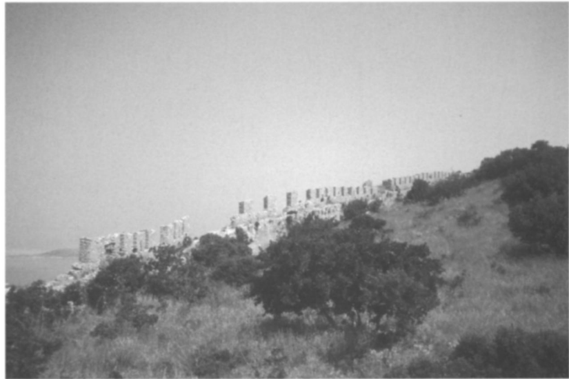
Figure II.13. Portion of the western circuit of the outer fortress, from the southeast
