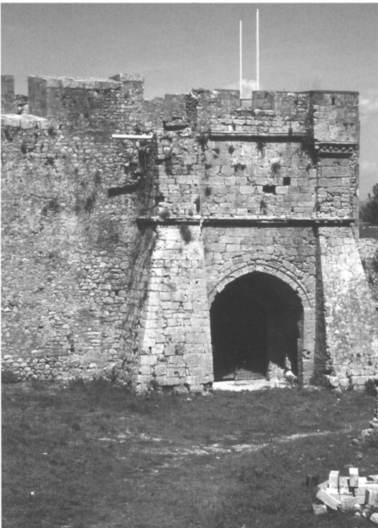
Figure III.8. Main (northeastern) entrance to Anavarin-i cedid
