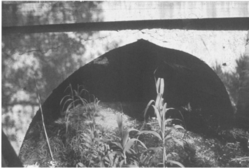
Figure 3.22. Arch of an old bridge over the Selas River near Romanou
