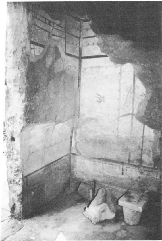
Figure 2.16 Casa del Fabbro, Pompeii, room 4. One of a series of small cubicula along the side of the atrium (see Fig. 3.24), the left-hand wall incorporates a recess for a bed. The decorative scheme is simple but elegant, with panels demarcated by plain borders, and golden motifs (griffins and cupids) floating in the centers.
