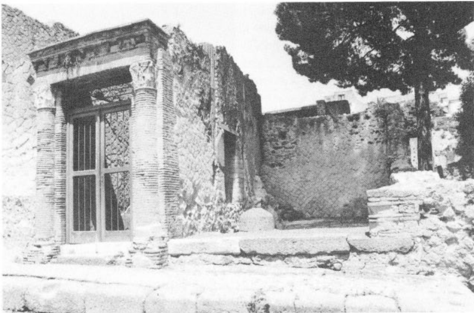
Figure 6.1 Casa del Gran Portale, Herculaneum, frontage. The narrow house-entrance is strongly marked by brick pillars (this distinctive feature gives the house its name). To its right is visible the wide threshold of a shop front. The shop no longer connects with the house (the doorway visible in its side wall is blocked), though it may have been linked in ownership and operation.
