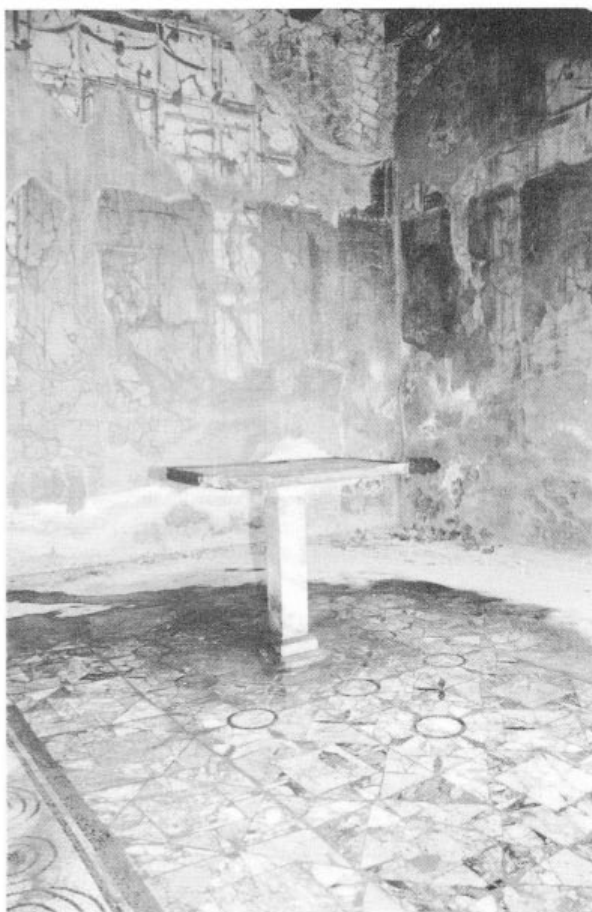
Figure 6.4 House V.II, Herculaneum, tablinum. The walls have rich fourth-style decoration, with mythological panels set against a red background, flanked by architectural vistas on a white background. The fine marble opus sectile floor forms a carpet in the center of spaces for couches (for a detail see Fig. 7.2). Note that the end wall of the tablinum in this small house is closed: the mythological painting is at the focus of the axial view from the entrance.
