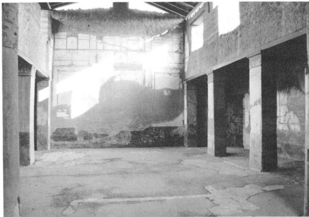
Figure 2.2 Casa dell'Atrio a mosaico, Herculaneum, view of oecus Aegyptius from atrium. The basilica-like construction permits a room of exceptional dimensions; the clerestory lighting enhances the sense of spacious elegance.
