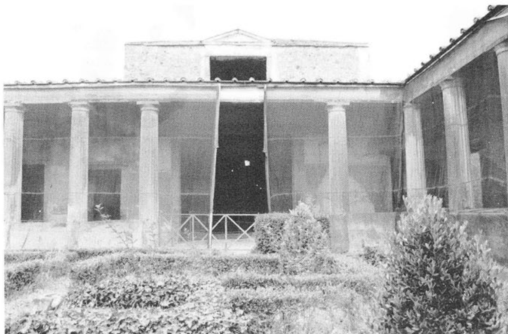
Figure 2.4 Casa del Menandro, Pompeii, view of peristyle, looking toward the largest reception room, marked by its wide opening on the peristyle, the double spacing of the columns, the high ceiling, and the pediment above a window for extra illumination.
