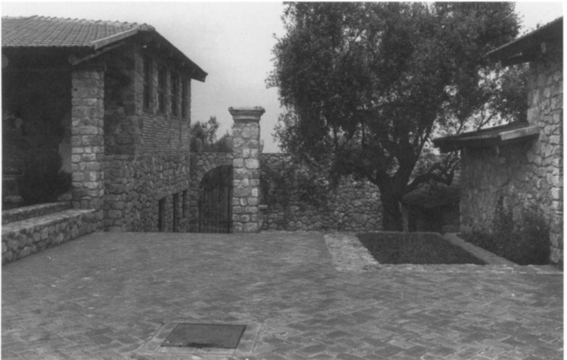
PLATE 5. V-D, museum courtyard and entrance, looking NW
