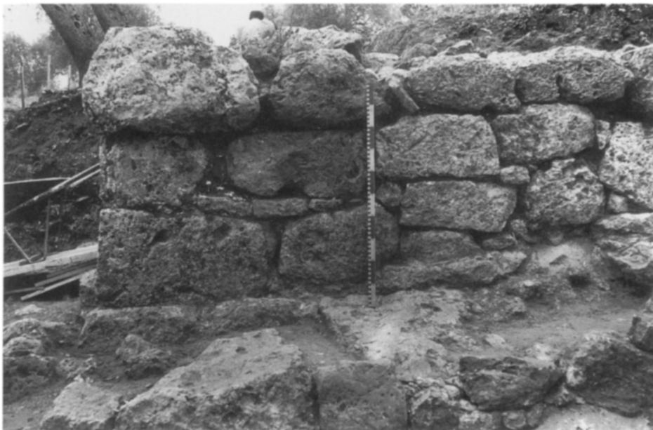
PLATE 59. East Block, Period 1.3: House of the Skeleton, north corner foundations, looking SE
