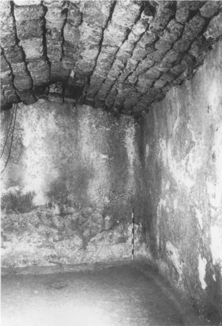
PLATE 68. East Block, Period 1.3: House of the Skeleton, cistern, interior
