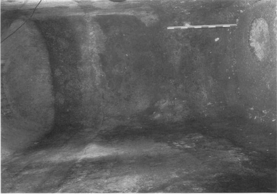
PLATE 22. East Block, Period 1.1: Northeast House, cistern, interior, looking SW
