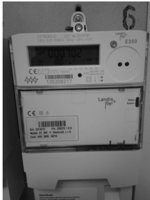
Figure 9.4 Close-up of the Smart Meter being used at the prototype location site.
