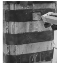
Figure 11. Failure pattern of column SP-2 (before stripping of bands).
