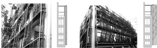
Shaded effect in the south side and diagrammatic cross section Shaded effect in the east side and diagrammatic cross section
