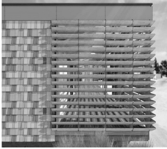
Figure 8. P11 with flood shutters.
