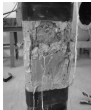
Figure 10. Failure pattern of column DP-5 (after stripping of bands).
