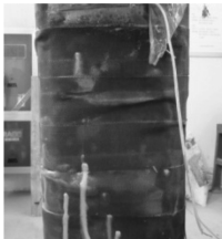
Figure 7. Failure pattern of column DP-4 (before stripping of bands).
