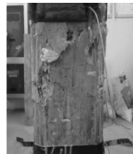
Figure 6. Failure pattern of column DP-3 (after stripping of bands).
