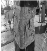
Figure 8. Failure pattern of column DP-4 (after stripping of bands).
