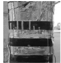
Figure 12. Failure pattern of column SP-2 (after stripping of bands).
