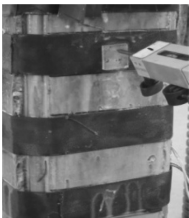
Figure 3. Failure pattern of column DP-2 (before stripping of bands).
