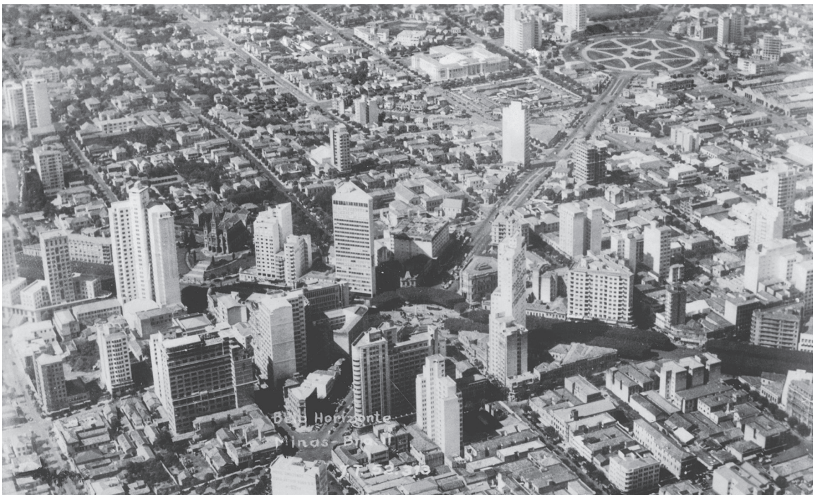
Figure 1.12. Aerial views of Belo Horizonte showing the densification of the grid in the late 1940s. Top, 1948; bottom, 1940s. Photos owned by author.
