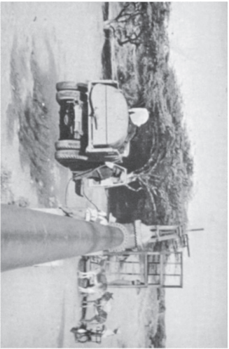
WATER, nearly five million gallons daily, reaches Pangana through this pipeline from a well. A truck is drawing supplies for the ham-
