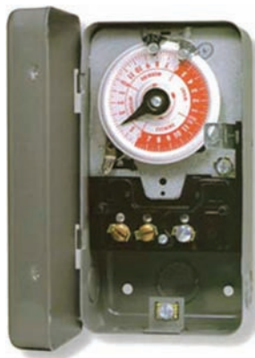
Figure 7-15 Synchronous clock timer.
