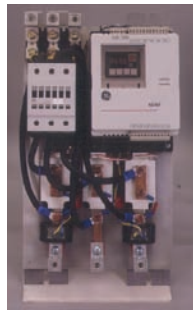
Solid-state reduced-voltage starter
