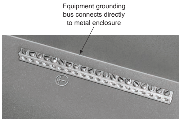
Figure 3-13 Equipment grounding bus.
