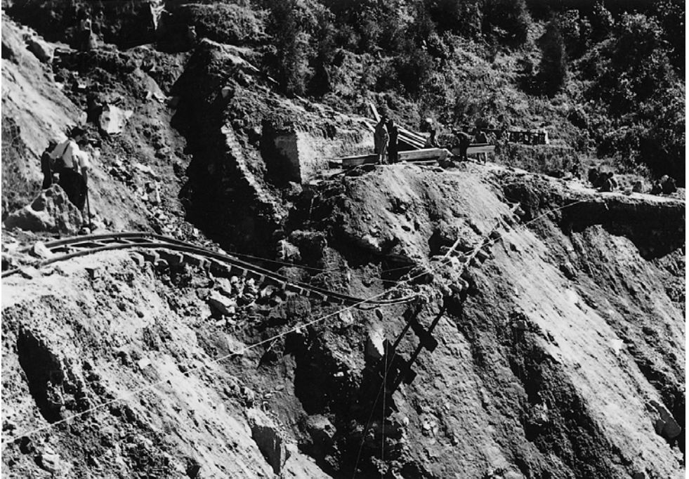
Figure 6.9 The famous Darjeeling narrow gauge railway closely follows the highway for much of its length. The October 1968 rainstorm caused almost total destruction with much of the line washed away and rolling stock precipitated hundreds of metres down the mountain side, November 1968.
