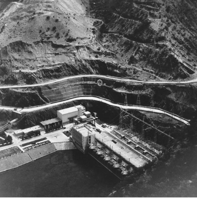
Figure 6.2 The Nurek Power Station, Tajikistan, on the Vakhsh River. The dam, located immediately off the right margin of the photograph, was built in part by volunteer Communist Youth labour and, at 300 metres, was reputed the highest rock- and earth-filled dam in the world. It is reported to have withstood an earthquake of Richter-scale 7.9 intensity. Photograph, July 1987.
