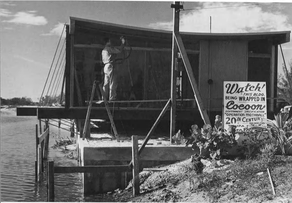
HEALY GUEST HOUSE (COCOON HOUSE), UNDER CONSTRUCTION
