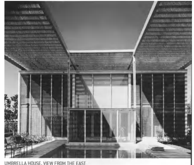
UMBRELLA HOUSE, VIEW FROM THE EAST
