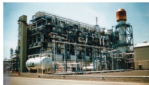
This plant in Tokuyama, Japan, passes ethane rapidly over a hot catalyst. The products are ethylene and hydrogen.
