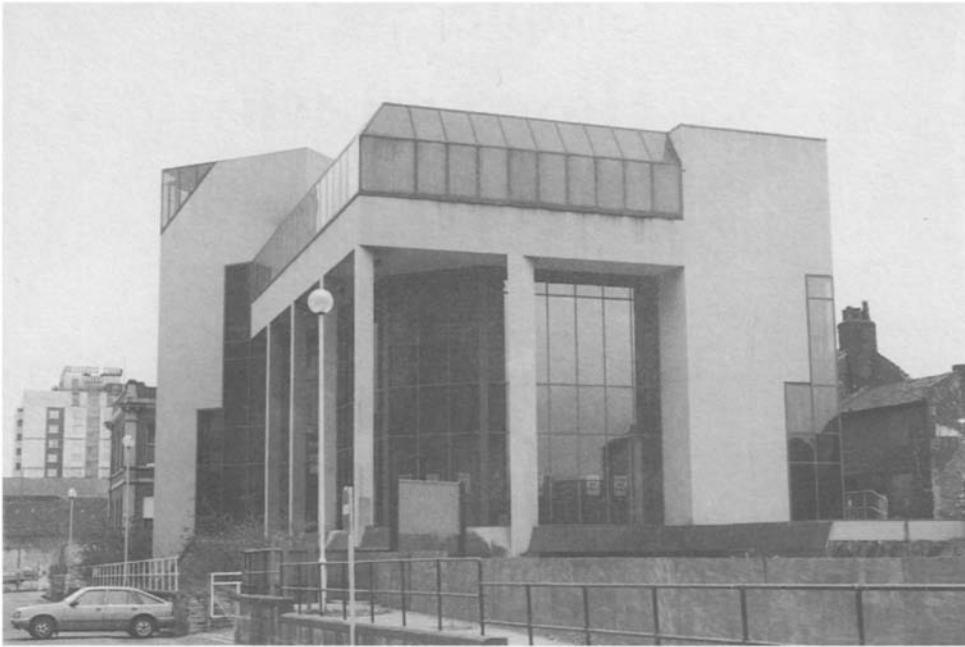
Figure 3.2 General view of a building clad with smooth faced stone panels possibly sandstone.
