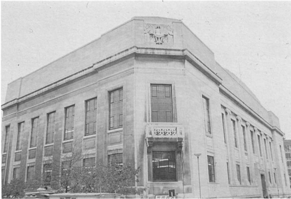
Figure 3.11 The elevation to the right of this public library faces south west while that to the left of the photograph faces north east and is heavily soiled.
