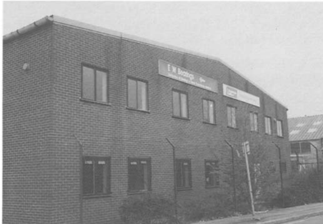
Figure 4.31 Staining at the joints of pre-formed metal verge cladding sections.
