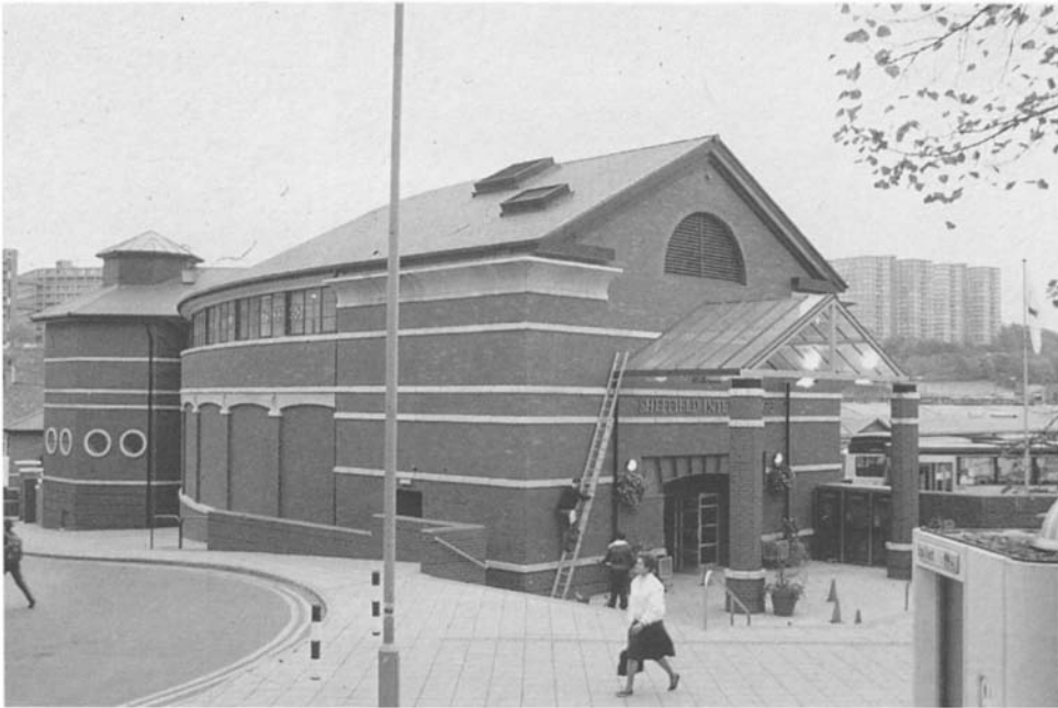
Figure 4.52 General view of building with cornice and string courses.
