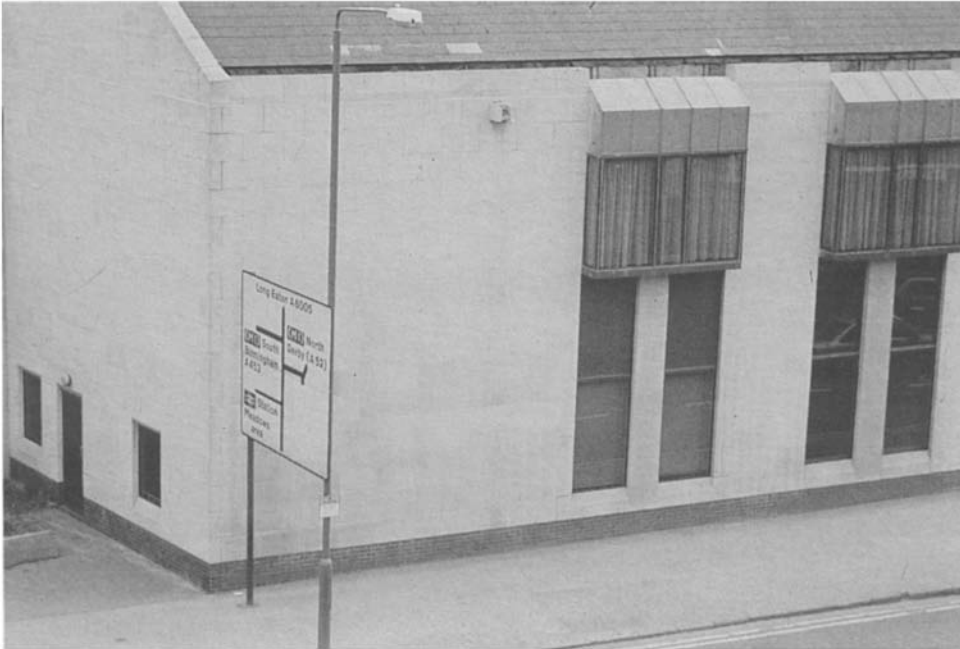
Figure 5.11 Cleaning the older building was slightly more successful but still did not return the façade to its original condition.
