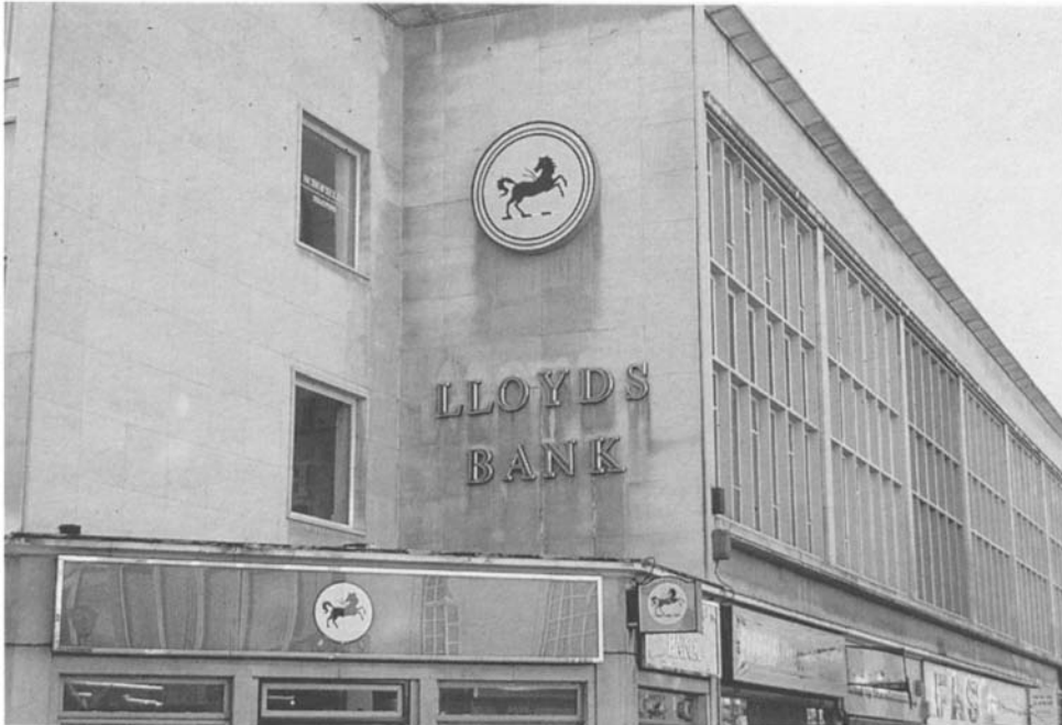
Figure 4.51 Logo and lettering fixed flush to stone cladding causing variable deposition and washing.
