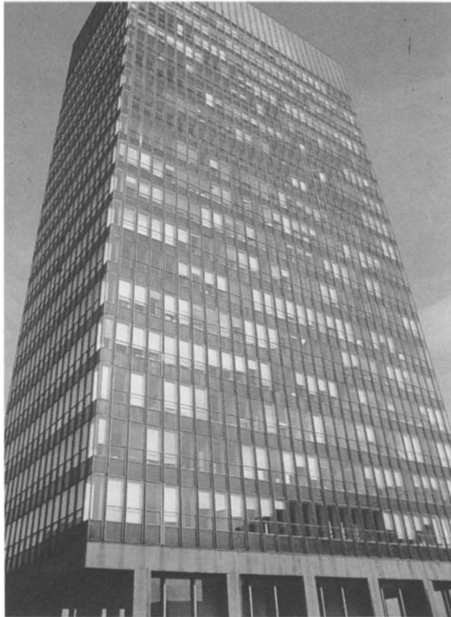
Figure 4.41 General view of multi-storey educational building clad with curtain walling with pronounced mullions.
