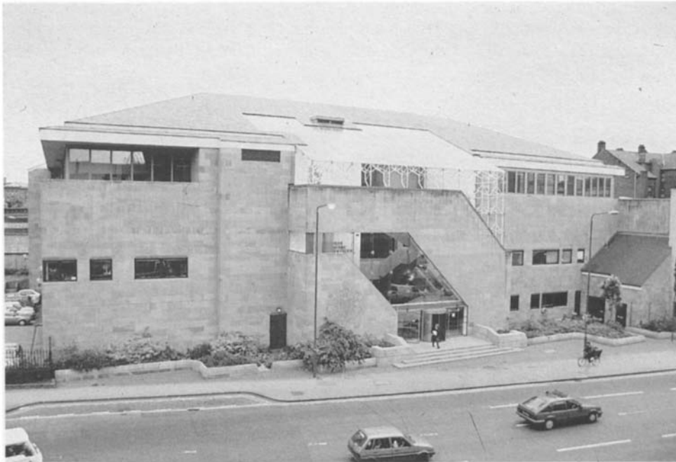
Figure 5.4 General view of stained law court building.
