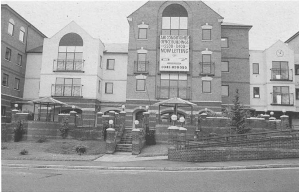
Figure 4.63 General view of a speculative office building adjacent to a busy motorway junction. Because of the difference in levels from the street and the entrance there is a considerable amount of staircases, ramps, planted areas, canopies, etc.
