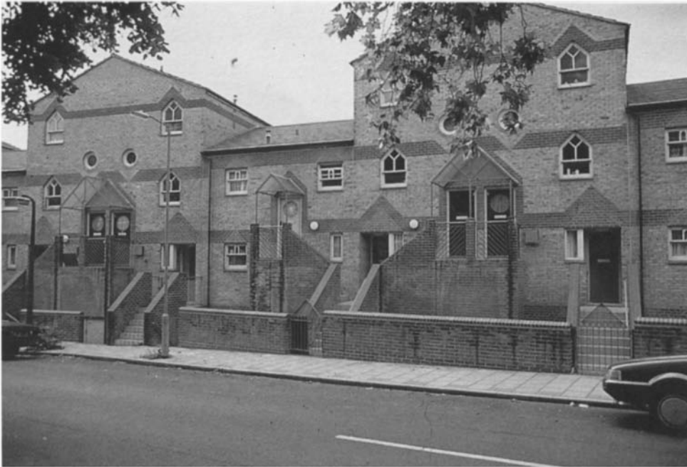
Figure 0.1 Elevation of housing development affected by premature staining.
