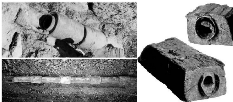
Fig. 8.7 Clay pipes ( left ) and oak pipes ( right ).
