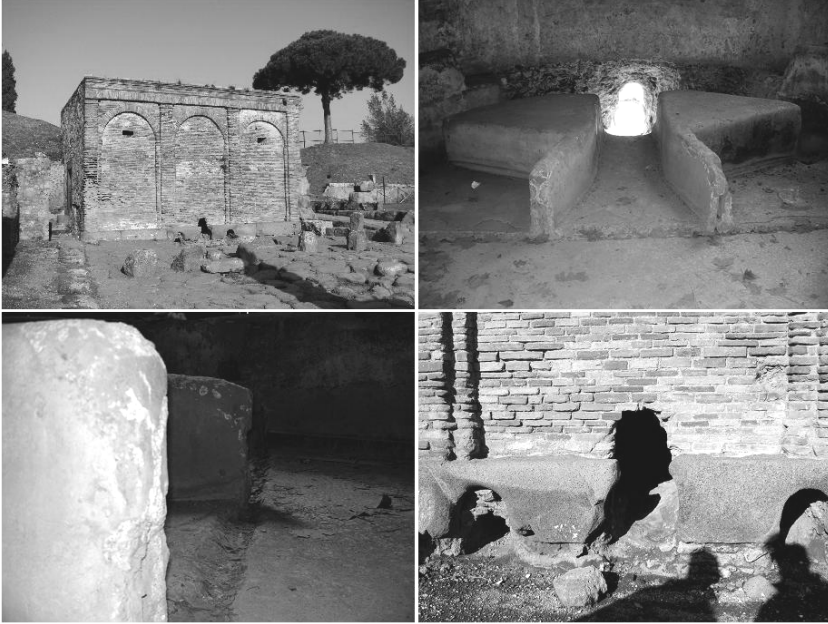
Fig. 8.4 The three-way distribution system at Pompeii.
