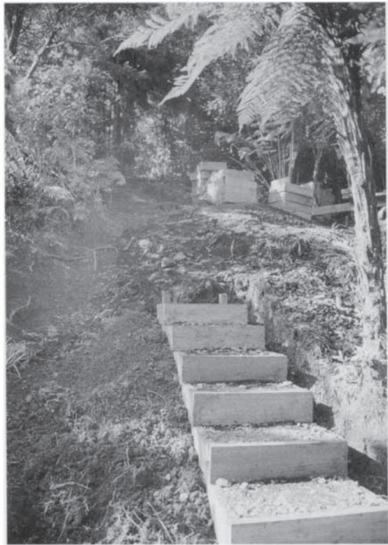
Plate 7.5: In order to minimise erosion caused by large visitor numbers in natural areas, substantial site and trail hardening may have to be undertaken as here in the Waitakere Regional Park, Auckland, New Zealand. However, what effects does such work have on the visitor experience and does the increased ease of access actually encourage yet more visitation?
