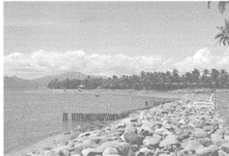
Plate 8.2: Denarau Island, Fiji. Modifying a mangrove swamp to build a resort complex has meant that erosion measures are necessary now the ecosystem has been changed.
