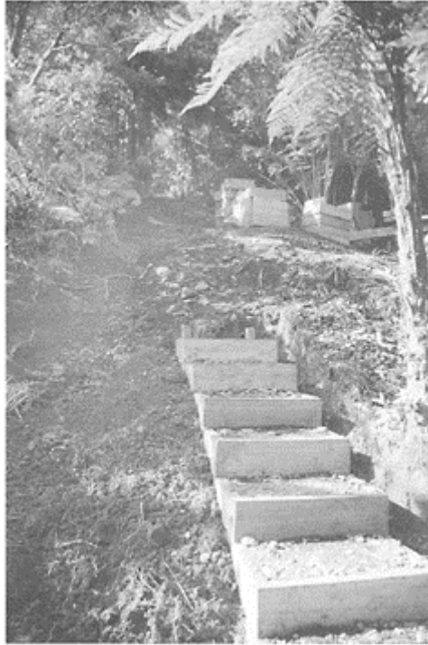
Plate 7.2: Waitakere Regional Park, Auckland, New Zealand. In order to minimise erosion caused by large visitor numbers in natural areas, substantial site and trail hardening may have to be undertaken, as here. However, what effect does such work have on the visitor experience and does the increased ease of access actually encourage more visitation?
