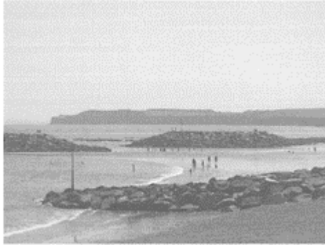
Plate 8.3: Sidmouth, England. Beach erosion protection.
