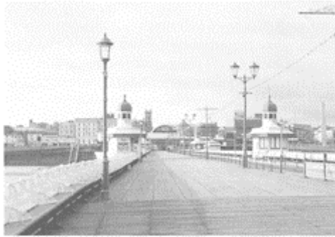
Plate 8.1: Blackpool Pier, England. The Victorians built piers to enable promenading as well as to represent humans dominating and taming nature (i.e. the coast and sea).
