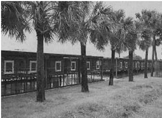
FIG 2.4 Outdoor facilities with a covered area to keep the food bowls and nest box dry can be used to breed birds in appropriate climates. The enclosure can be constructed over concrete pads with a drainage ditch to one side for ease of cleaning.
