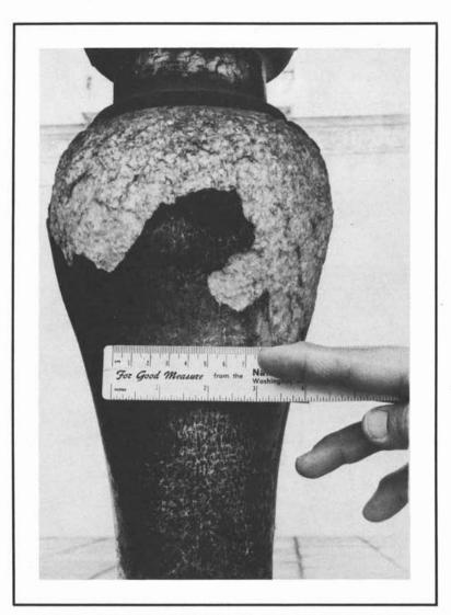
COVER Marble baluster in balustrade of the west patio, Pan American Union Building (completed 1910), Washington, District of Columbia. The black coating contains finegrained gypsum and is scaling off. Photograph by Deborah Dwornik, U.S. Geological Survey, 1984.
