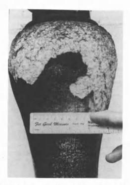
FIGURE 3 Gypsum alteration and spalling at the Pan American Union Building.
