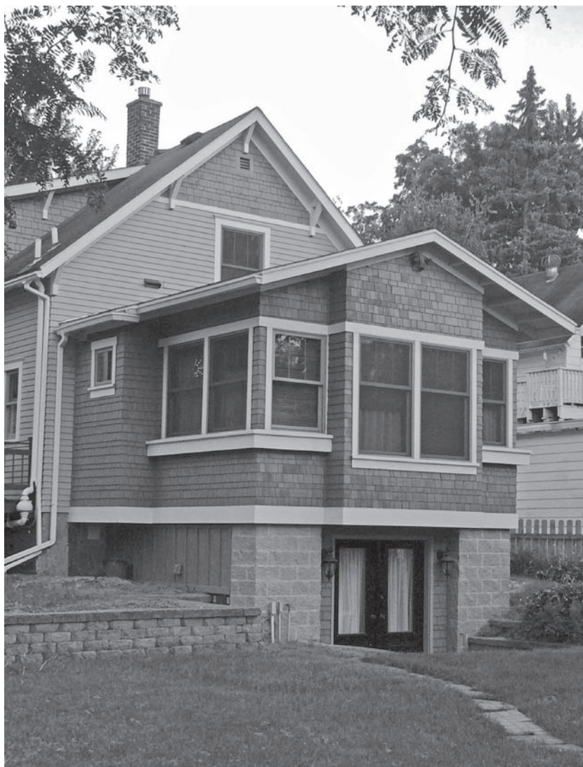
Figure 10-1 This residence was remodeled with a two-story rear addition providing a new bathroom, family room, and home office.
