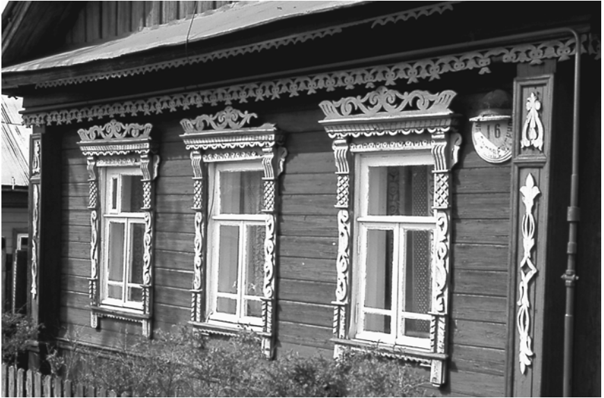
12-5. On this cottage in Kostroma, Russia the elaborately carved window surrounds are supplemented by other decorative wooden carvings (photo by the author, 1997).
