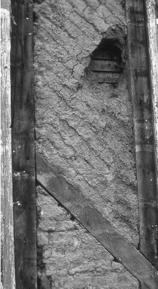
6-10. Layers of mud nogging placed at an angle determined by the cross-brace of the timber frame. The mud was added in rows with each row allowed to dry before the next row was applied. Ruins of a house near Columbia, Missouri (photo by the author, 1980).
