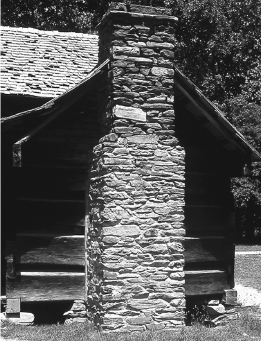
11-2. Good example of an exterior stone chimney attached to a log house. A variety of boulders and flat fieldstones have been used. A lime mortar binds the stone. Note also the large boulders upon which the sills of the house rest. Located in Cades Cove, TN (photo by the author, 1972).
