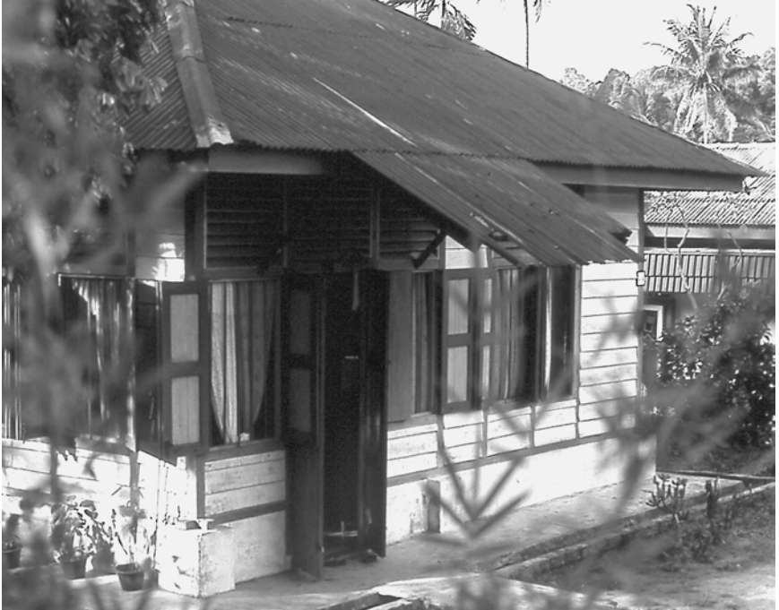
10-4. The oversized projection of the corrugated iron roof helps to deflect the heavy tropical downpours from the doorway of this dwelling in Johore, Malaysia (photo by the author, 1980).
