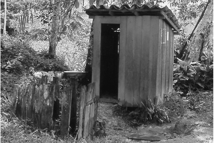
3-1. The well and the privy are conveniently located adjacent to one another. Unfortunately, their proximity is an invitation to contamination of the water supply. A cobocolo farmstead in the Amazonian rain forest near Belem, Brazil (photo by the author, 1963).
