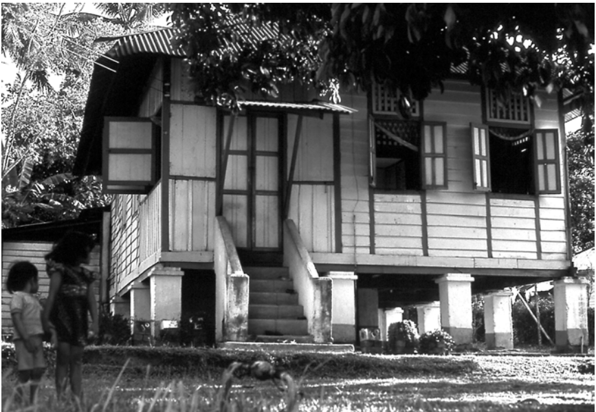
7-14. This stilt house in Johore, Malaysia is raised on sturdy cement pillars. Note also the many window openings that provide ventilation in this constantly warm environment (photo by the author, 1980).
