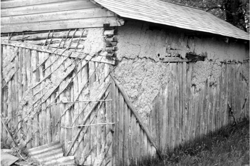
6-4. Both vertical and horizontal round logs form the walls of this Ukrainian house near Senkiw, Manitoba. Light willow sticks are attached to the logs to act as an anchor for the mud daub, much of which has already disappeared (photo by the author, 1983).
