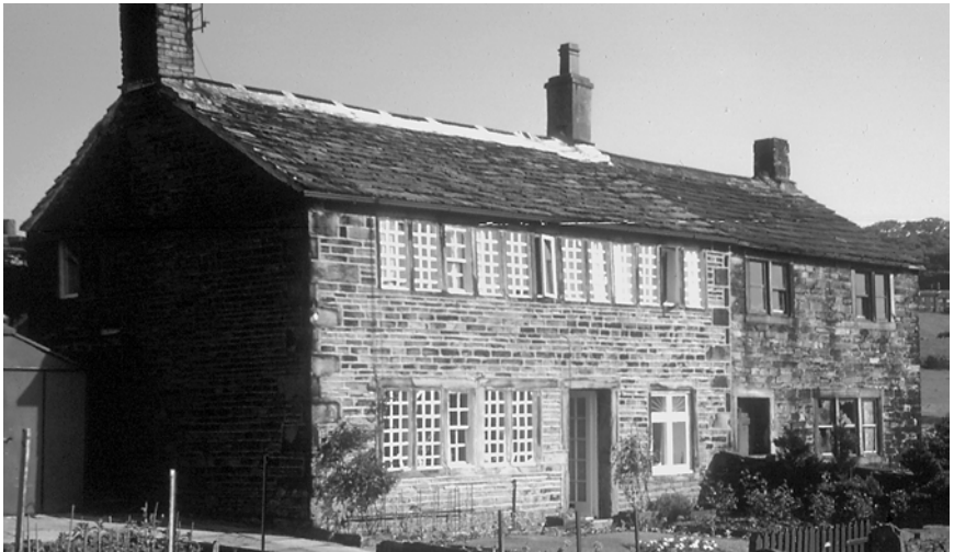
4-1. A weaver's house, Almondbury, Yorkshire, UK. The large number of windows documents the 18th-century conversion of the dwelling to enable weavers to work with enhanced natural lighting (photo by the author, 1967).
