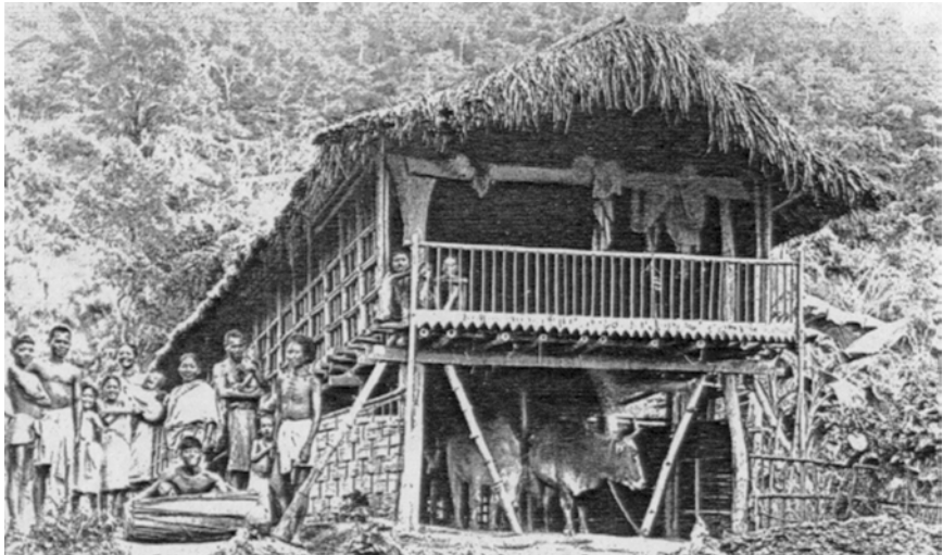
13-5. Stilt-supported longhouse from Assam, India. Note the cattle tethered on the ground below the house platform (from Scherman 1915, tafel 10).
