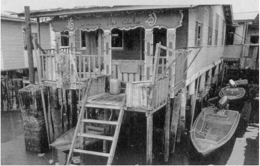
9-4. Stilt house in Brunei in which modern concrete pillars are replacing traditional wooden ones. Nevertheless, the character of the structure is not much altered because the posts, although different in material, are quite similar in form (from Hansen 1995, 34. Courtesy of Eric Hansen/Saudi Aramco World/PADIA).
