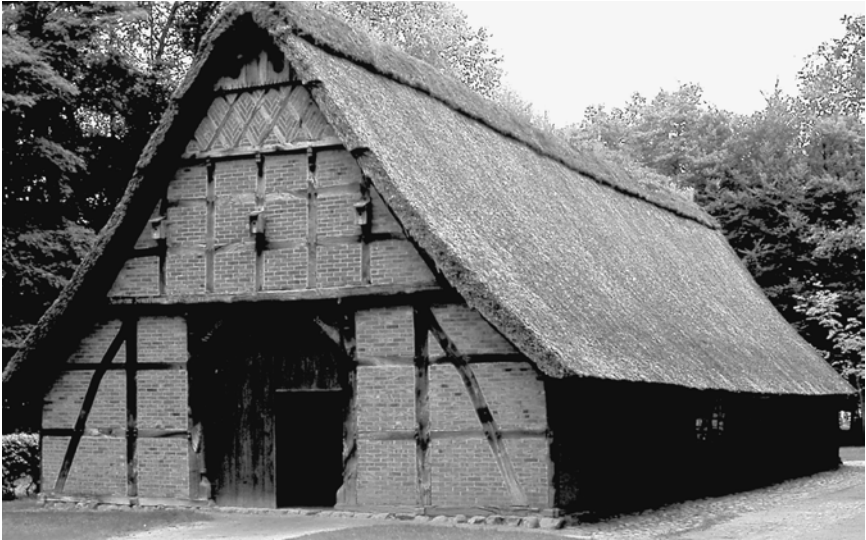
2-6. This brick and half-timber Hallenhaus is preserved in the Cloppenburg Open-Air Museum, Germany. Note the extra layer of thatch along the ridge and the bellcast of the eaves, both features to provide maximum rain protection (photo by the author, 1982).
