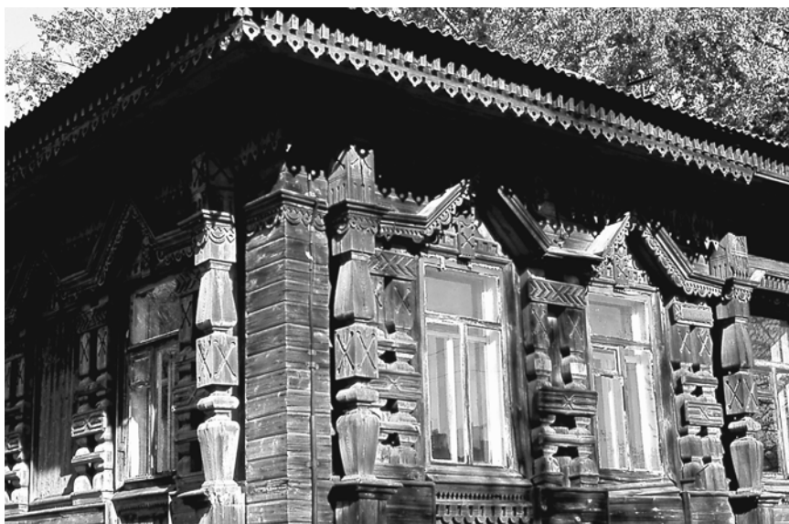
12-4 An unpainted, but elaborately carved, izba in Uglich, Russia. Note the matching eave dentils and the carving under the windows (photo by the author, 1997).
