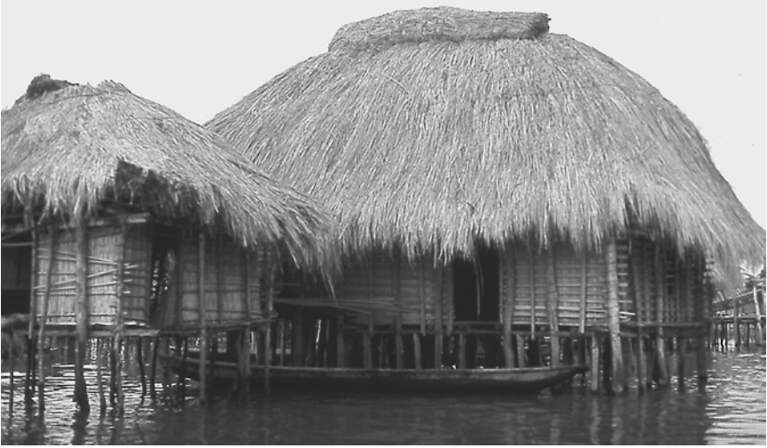
8-8. A thatched hipped roof is typical of many structures in the Ganvie lagoon, Benin. Note the extra layers of thatch along the ridge to provide maximum rain protection at the most vulnerable area (photo by the author, 1980).
