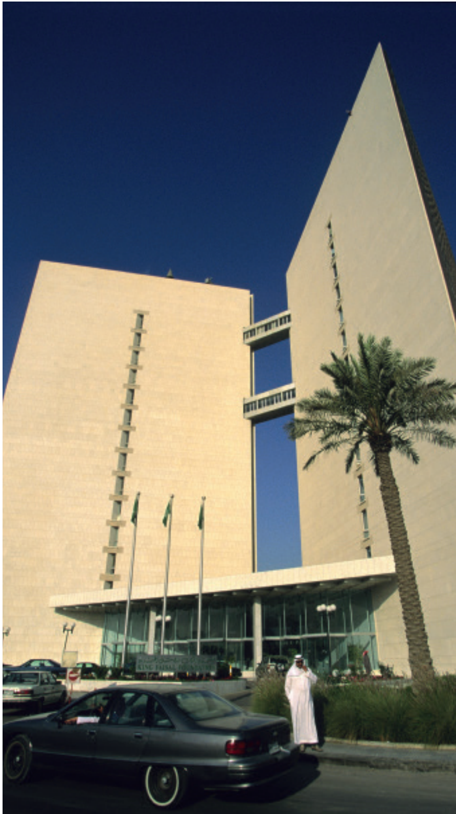
LEFT Kenzo Tange Associates, King Faisal Foundation headquarters, Riyadh, Saudi Arabia, 1984
