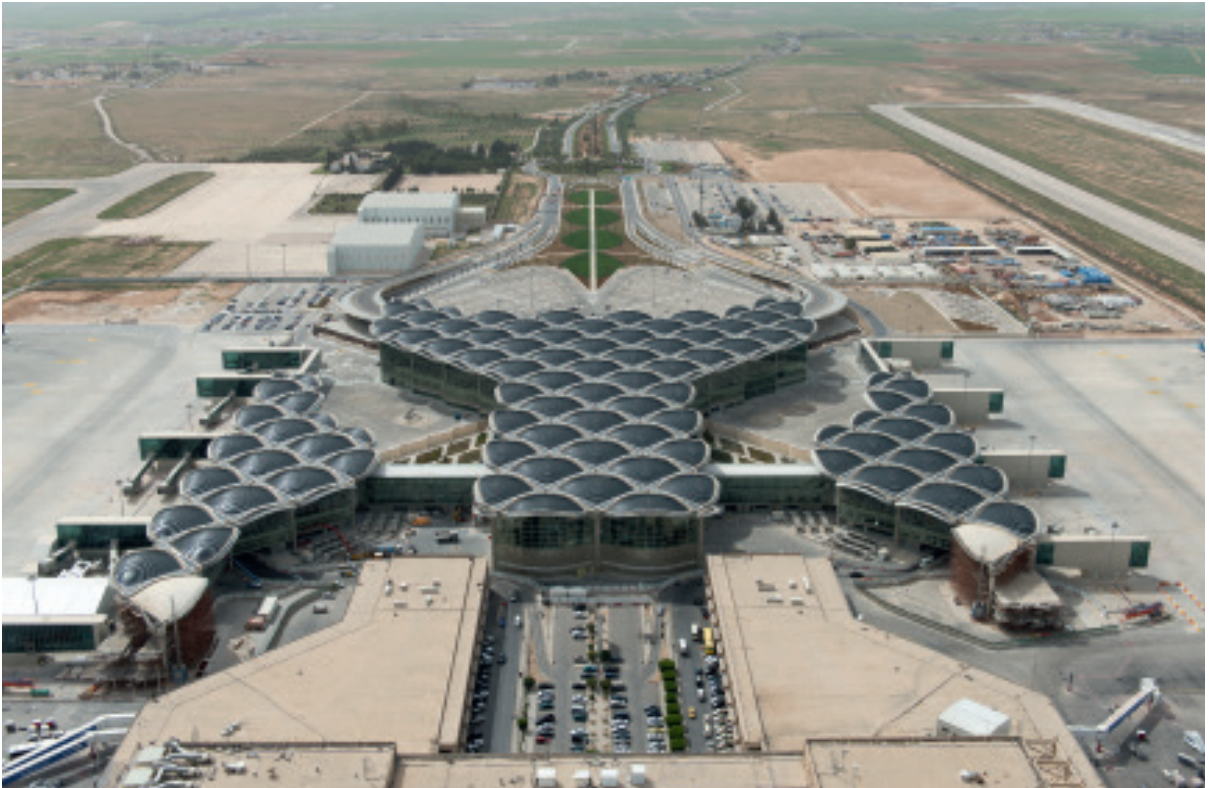
ABOVE Foster + Partners, Queen Alia International Airport, Amman, Jordan, 2005 The structural system is itself a geometrical structure, like the skeleton of a living creature.
