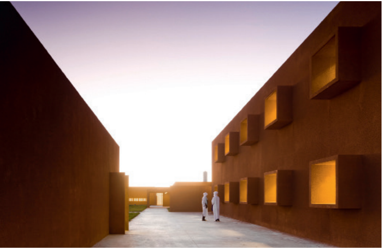
ABOVE Driss Kettani with Mohamed Amine Siana and Saad El Kabbaj, École Supérieure de Technologie de Guelmim, Guelmim, Morocco, 2011 A project that explores both contextualism and sustainability in order to generate human-scale spaces with passive thermal comfort in the hot south of Morocco. It also demonstrates that sustainability can be generated in situ without resorting to foreign materials.
