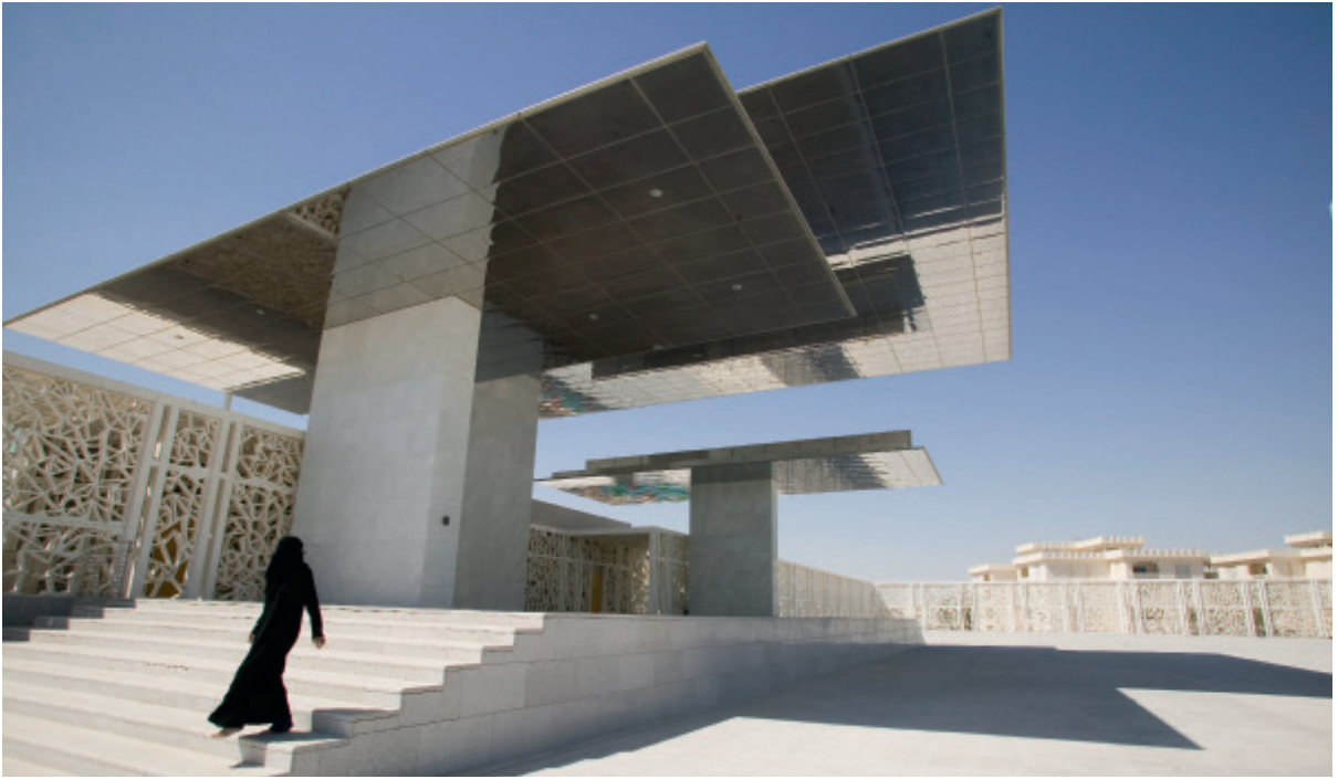
ABOVE Qatar Foundation, Education City, Doha, Qatar, 1995 Light explored through solar panels integrated in architectural design to provide energy.
