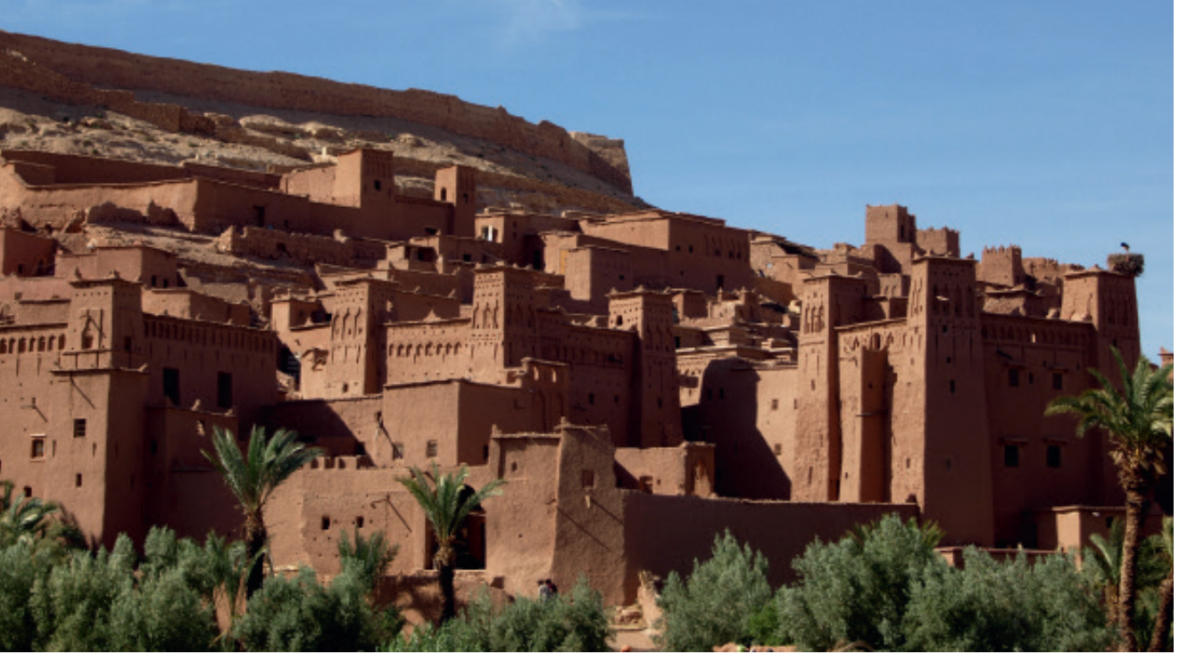
ABOVE Ksar of Ait-Ben-Haddou, Morocco, 17th century An example of how climate and physical context considerations have given local architecture its character.
