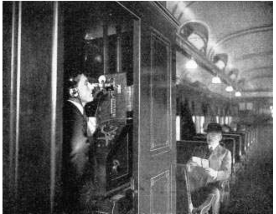
Fig. 14.2 Wireless telephony on the train. The installation is in a small cabin about 2 by 4 feet at one end of the car.
