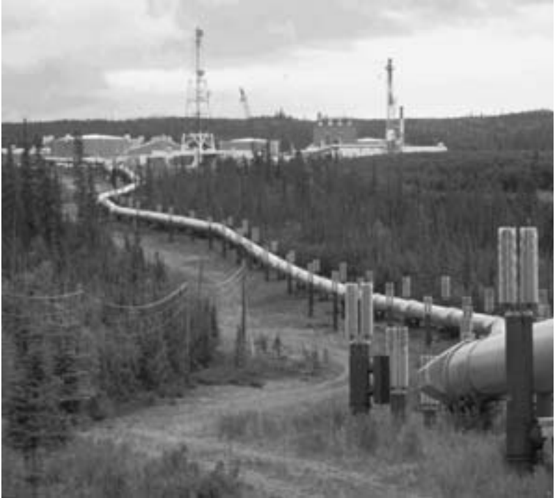
The Trans-Alaska pipeline begins in Prudhoe Bay on Alaska's North Slope and ends 800 miles (1,280 kilometers) away in Valdez, the northernmost ice-free port in North America. The pipeline started transporting oil in 1977, and over 13 billion barrels of oil have already moved through its pipes.
