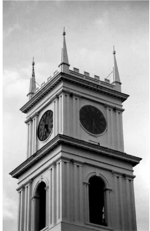
Figure 4. Four lightning rods on top of old Whaling Church, Edgartown, Massachusetts (photograph courtesy of William Waterway).
