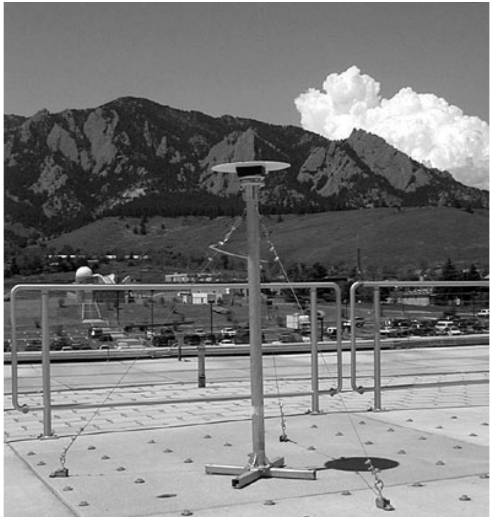
Figure 14. GPS receiver placement on top of FSL's new office building, the David Skaggs Research Center.
