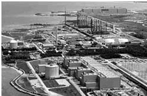
Figure 2. Bruce Heavy Water Plant in Ontario, Canada (Toronto Star, Online Edition, Dec. 2, 2003).
