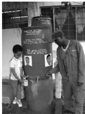
Figure 4. The EnDeCo Institutional Defluoridator. It can be made at any desired capacity, normally in the range 20–160 m 3 for a raw water fluoride of 5 mg/L.
