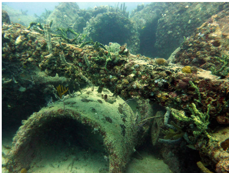
Reef Coasts, Figure 6 Construction debris used to build an artificial reef offshore southeast Florida, USA. This man-made reef structure was constructed by placing steel rails and circular concrete culverts within a specific zoned area on a sandy seafloor landward of the Florida Reef Tract. Over time, marine organisms, such as sponges and scleractinian coral colonies, utilized the artificial reef substrates to adhere and grow, just as they would on natural reefs. Colonization along the steel rail transecting the photo center shows a wide range of biological marine life upon its surface (photo: Christopher Makowski).
