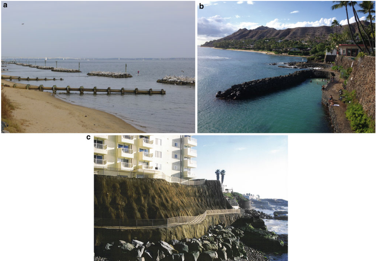
Coastal Engineering, Figure 1 Examples of shoreline protection: (a) Bay Ridge Beach, Chesapeake Bay, MD, USA – timber groin and rock berm breakwater system protecting recreational beach and coastal roadway (photo: Louise Wallendorf). (b) Shangri-La Center for Islamic Art, Oahu, Hawaii, USA – breakwater creating small boat refuge and beach (photo: Rob Walker). (c) San Diego, CA, USA – community bank protection and public walkway using naturally finished concrete seawall and a rock revetment – extreme wave climate (photo: Walter Crampton, TerraCosta Consulting Group).
