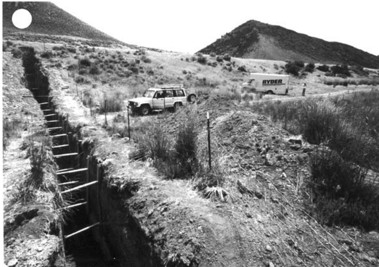
Figure 2A.22: Single-slot trench excavated into the face and toe of an 8 m-high normal fault scarp, eastern Bear Lake fault zone, Utah. Note the tops of 2.1 m-high hydraulic aluminum shores visible in the trench.
