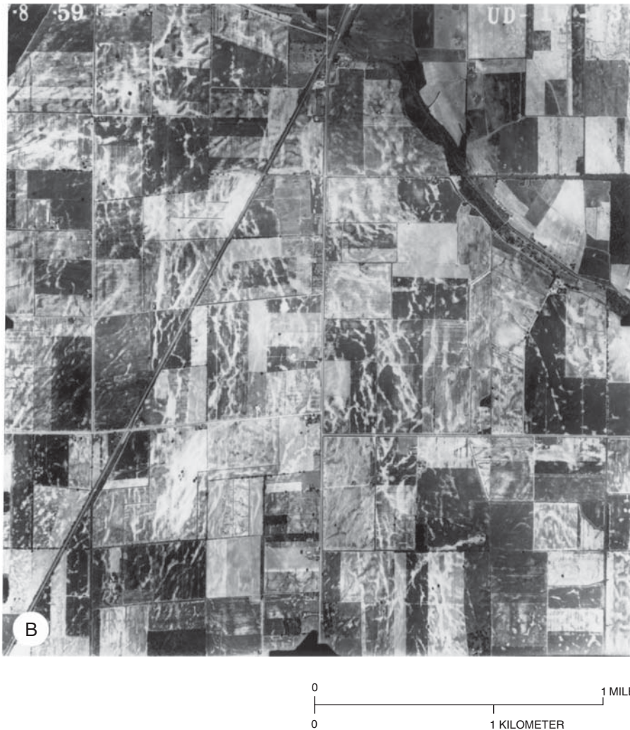
Figure 7.15: Aerial photos that show long fissures (dikes) through which sand vented (light-colored linear features) and also individual sand blows (light-colored spots) formed by liquefaction during the 1811–1812 New Madrid earthquakes. (A) A portion of the Manila, Arkansas, 7.5-min orthophoto quadrangle. Fissuring and venting took place in braid-bar deposits of latest Pleistocene age and in younger Holocene point-bar sediments. Note how fissures formed parallel to the scrolls of point-bar deposits. Note also the abundance of fissures in the upper part of the right side of the photo. These fissures of lateral spreading origin have formed near a break in slope, where the terrace that is underlain by braid-bar deposits is adjacent to the slightly lower floodplain level of point-bar deposits. Isolated sand blows in upper left formed by hydraulic fracturing. (B) Aerial photo taken about 40-km north of part (A). Extensive fissuring and venting in braid-bar deposits of latest Pleistocene age. Cap thickness (about 6 m) is relatively uniform. Topographic relief is about 1 m throughout the region. Note severe fissuring over a width of at least 3 km. Long fissures probably formed by surface oscillations, because relief seems too low for lateral spreading.
