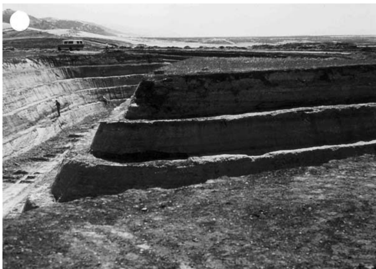
Figure 2A.26: Photographs of an early double-benched trench excavated by bulldozer, at the site of the proposed Point Conception (California) liquefied natural gas terminal. Note person at far left for scale. The project was proposed in 1972, but by the time site suitability studies were completed in 1980 (including seismic hazard studies; Rice et al. , 1981), oil prices had fallen so much as to make the project uneconomic, and it was abandoned (photograph courtesy of T. K. Rockwell).
