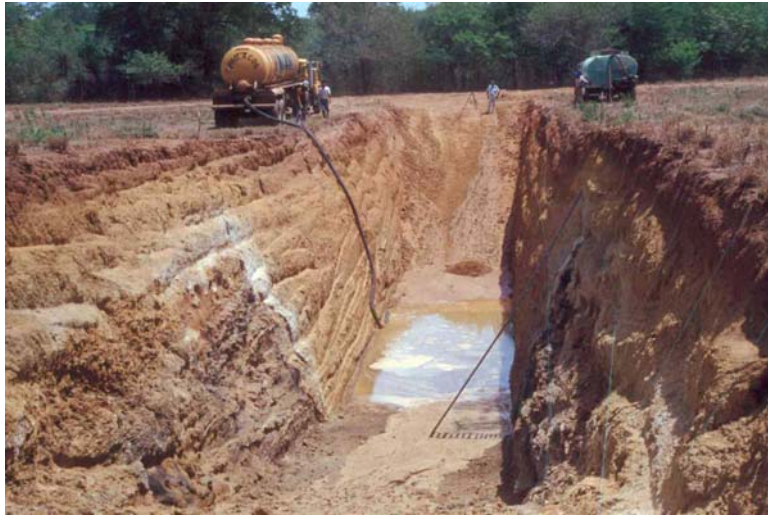
Figure 2A.30: “Venezuelan-style” trench dug by Audemard (2005). Trench is 90 m long, 8 m deep, 8 m wide at top, 4 m wide at bottom; excavated volume is ca. 3600 m 3 . Note the steep sidewalls, lack of benches, and string reference grid on right wall. To make contacts more visible the walls were wetted by the water truck at right; at left a vacuum truck is pumping out the collected water in the trench bottom. Photo courtesy of Franck Audemard.
