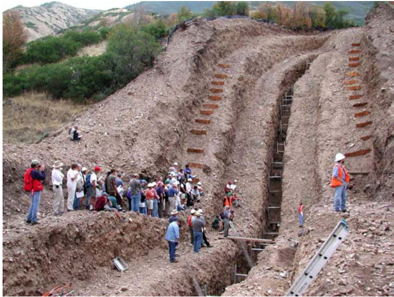
Figure 2A.19: A large benched trench across a 23 m-high normal fault scarp on the Wasatch fault zone at Mapleton, Utah. Note the deep inner slot which is shored, and small vertical boards on the first bench, to assist in climbing up the trench. Preliminary results are described by Olig et al. (2005).
