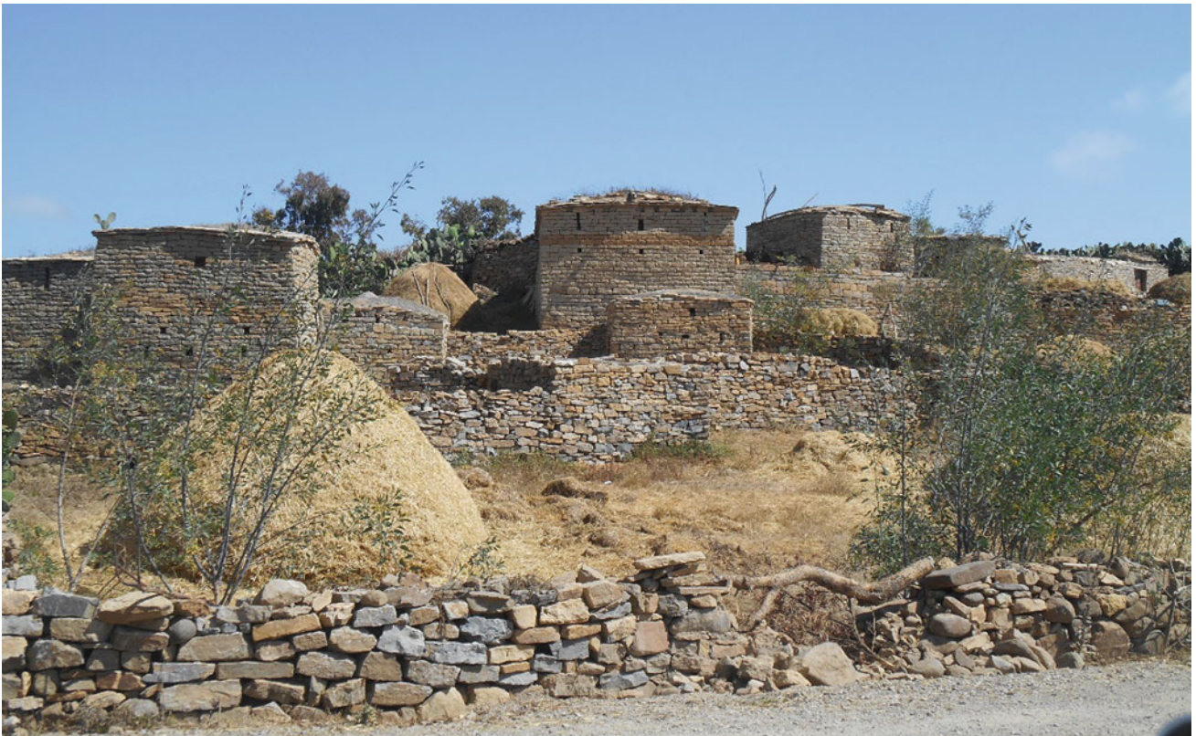
Fig. 4.8 Hamlet near to the escarpment, south of Makale, with “dry rock” walls built from Jurassic limestone ( Photo Varet 2005 )
