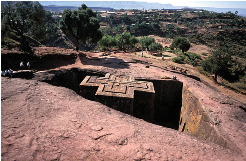
Fig. 3.3 Lalibella Coptic church dug in the ignimbrite of the Ethiopian plateau covering the trap basalts as observed in the plans behind (Source www.boundless.com )
