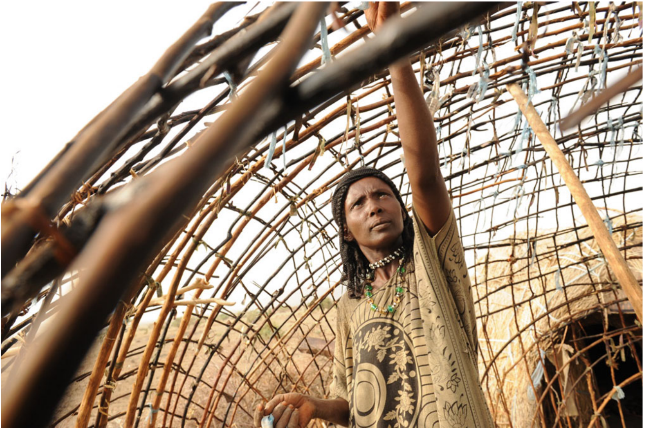
Fig. 2.18 Building the wood framework for a house ( Photo credit Ismail Ali Gardo)
