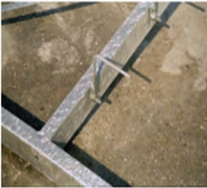
Figure 7.7 Basic arrangement of a bonded fixing. The bonding pad envelops the anchor. (Courtesy of G. Jones.)
