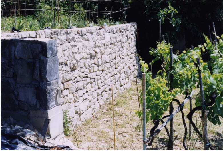
Fig. 10. Rebuilt wall bordering a terraced area near S. Croce, Trieste municipality (source: Antonini M.)
