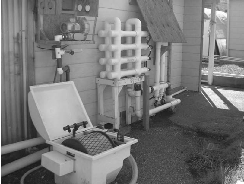
Figure 5.3 Picture shows a drum filter to remove solid material from the water line, two UV light sterilizers (mounted on wall), and an air blower for supplying air to each tank. The large UV unit contains 8 tubes (40 W each) and the small unit under the plywood contains two tubes (200 W each). These components are for the tank array in Figure 5.2.
