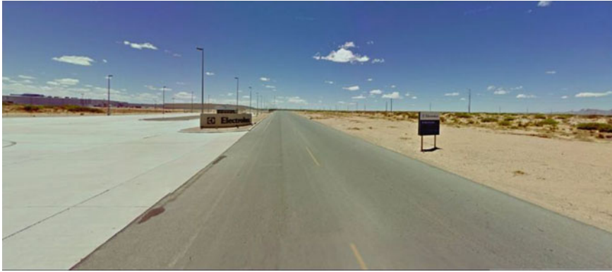
Photo 2.10 Access road to Electrolux Plant, view from North. Source Image capture: Apr 2009 @ 2014 Google
