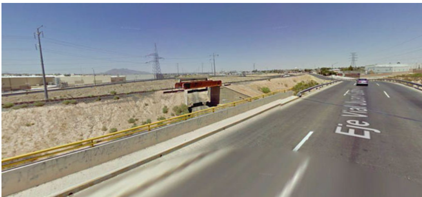
Photo 2.4 Orange bridge, view from the south. Source Image capture: Apr 2009 @ 2014 Google
