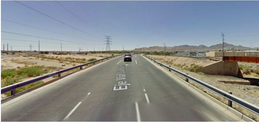
Photo 2.5 Orange bridge, view from the north. Source Image capture: Apr 2009 @ 2014 Google
