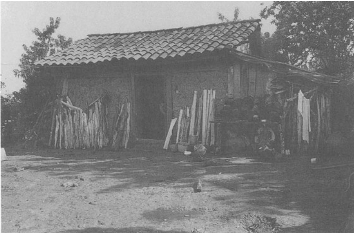
Figure 5-2. Zinacantan, Chiapas, Mexico (MS001), showing two house types. Top, “Chukal Na” (thatch roof, wattle-and-daub walls); bottom, Ladino style (tile roof, adobe walls). Top photograph is courtesy of Frank Cancian and is from Vogt (1969: Figure 21). Reprinted with permission of Evon Z. Vogt and Harvard University Press. Copyright © 1969 by the President and Fellows of Harvard College. Bottom photograph courtesy of Frank Cancian.
