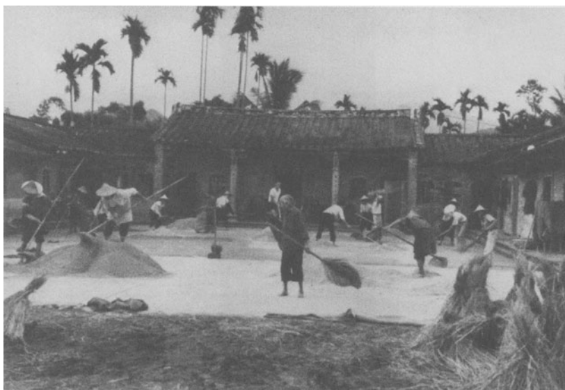
Figure 3-2. CH019, Yen liao (CH05), “U”-shaped courtyard formed by the central shrine room (facing), and two wings of living/sleeping rooms. From Cohen (1976: 107). Reproduced with permission of Myron L. Cohen and Columbia University Press.
